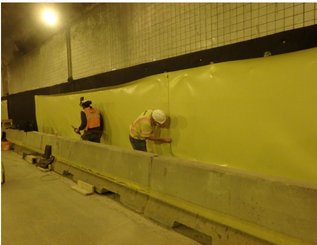
Fig. 5: PVC membrane installation - Specialist contractor Schneider-Moran is installing the first sections of waterproofing in the eastbound tunnel on the lower sections of tunnel wall.
