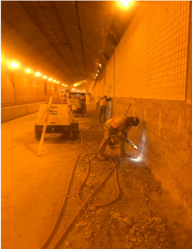
Fig. 4: Demolition 1 - The barriers at the side of the eastbound tunnel were removed so that the new waterproofing system could be installed.
