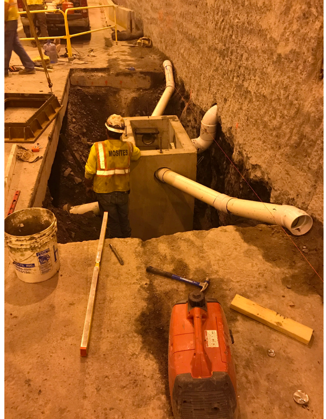
Fig. 2: Drainage installation - The new 'umbrella' waterproofing in the eastbound tunnel will be directed into the existing system beneath the tunnel.
