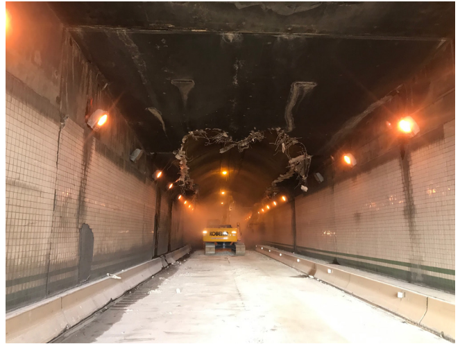
Fig. 3a: Work underway in Eastbound - Mosites has removed the ceiling and the barriers at either side of the tunnel. Each weekend, the tunnel must be reopened to traffic.
