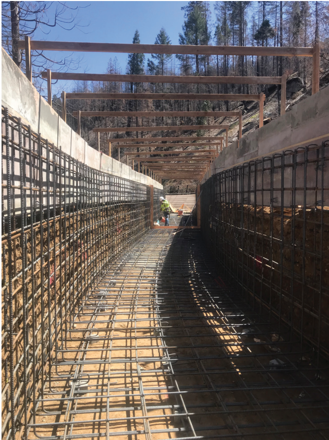
Fig. 3: Canal before shotcrete
