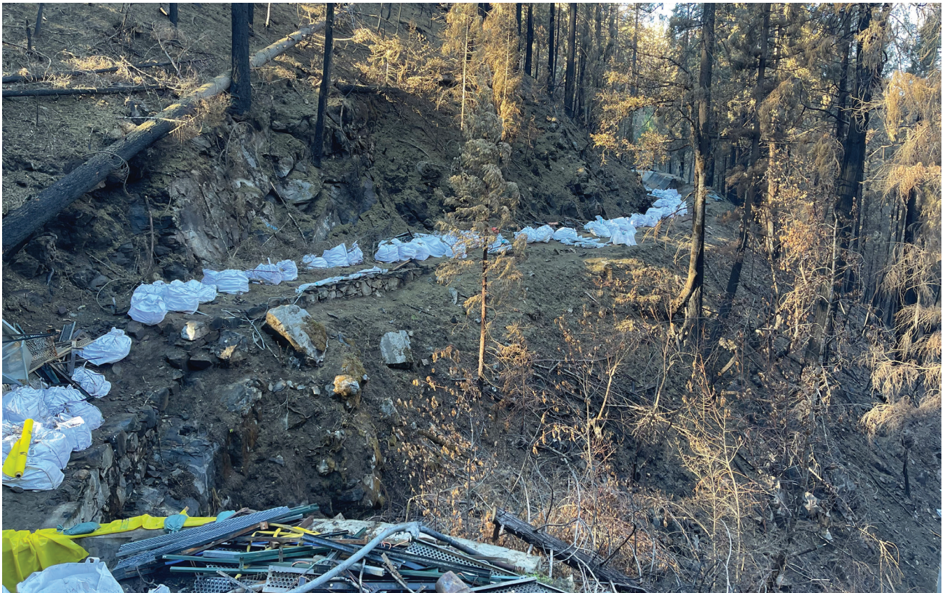
Fig. 1: Before shotcreting of the flume
