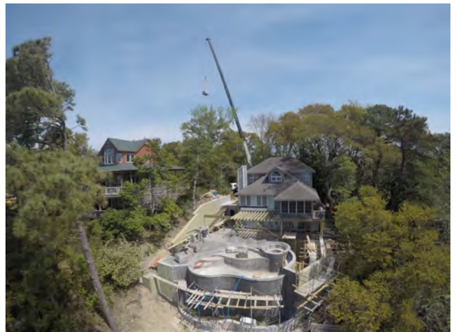
Fig. 11: Pallets of stone moved via crane due to site accessibility issues.
