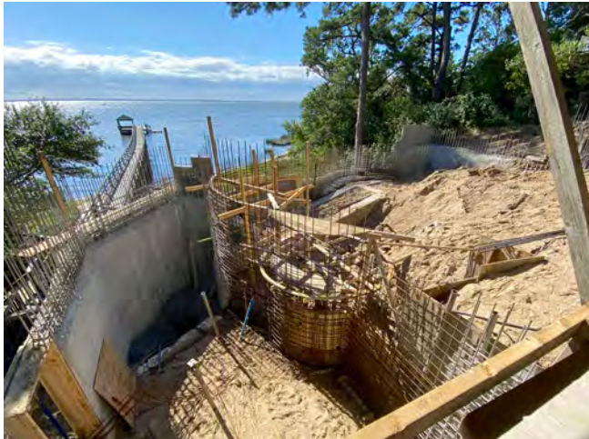
Fig. 8: View of curved forms and rebar for the bottom-up approach.
