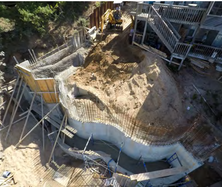
Fig.7: Backfilling shotcreted walls.
