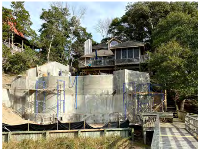
Fig. 10: Finished shotcrete view of the vanishing edge.
