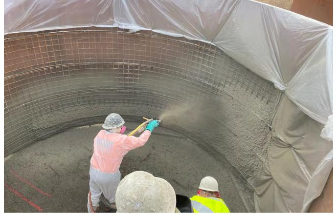
Fig. 3: Mock-up: Shotcrete placement.
