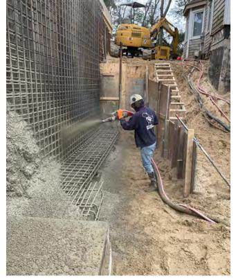
Fig. 9: ACI-Certified Nozzleman shooting wet-mix on the 21 ft retaining wall.
