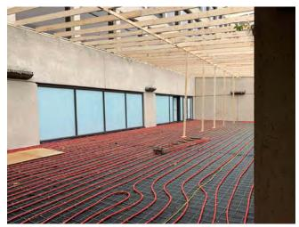
Fig. 11: Concrete slab with heating piping for melting ice and snow.
