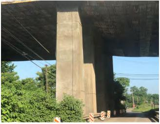
Fig. 13: Four gunned and completely finished piers in the Glenfield Borough section of the project.
