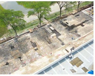
Fig. 6: Overview of roof slab with full depth repair areas apparent.
