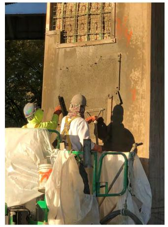
Fig. 11: The cutting-down and finishing work has to be done in a timely manner. Working out of man lifts necessitates a stop and go procedure.
