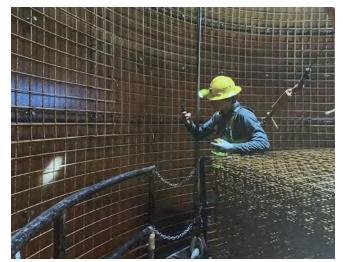
Fig. 7: Inspection to ensure the correct overlap of WWR.
