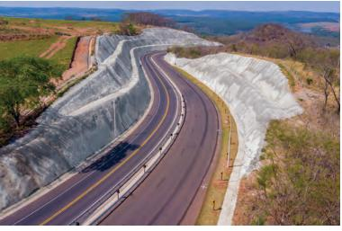
Fig. 10: Slope after shotcrete application.
