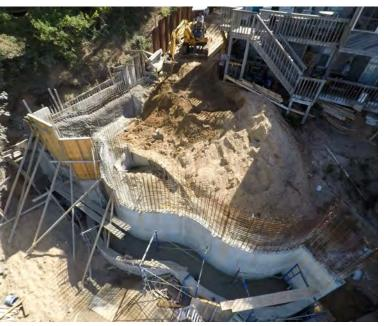
Fig.7: Backfilling shotcreted walls.
