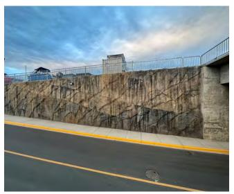
Fig. 4: Architectural rock finish—additional view showcasing coloring.
