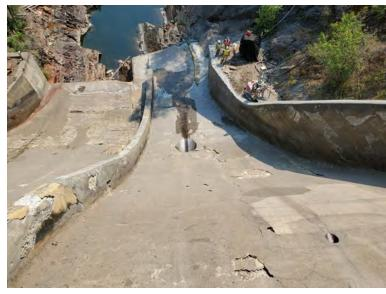
Fig. 5: Left spillway at Moyie Dam showing old shotcrete, 2021.
