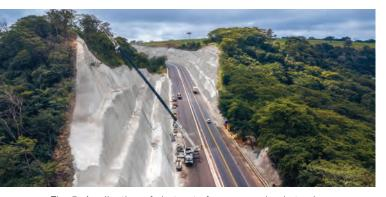
Fig. 5: Application of shotcrete from a man basket using a crane.
