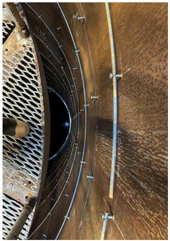
Fig. 6: Detail of #4 bar tied to the studs.
