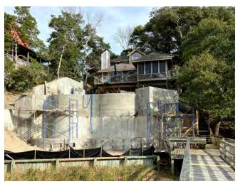
Fig. 10: Finished shotcrete view of the vanishing edge.
