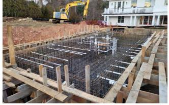
Fig. 3: Rigid forming, plumbing, and reinforcing steel installation.
