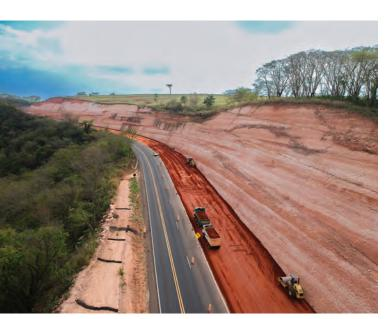
Fig. 3: Excavation and slope process for highway expansion.
