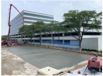
Fig. 9: Replacement roof slab.
