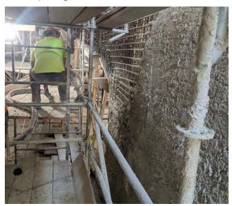
Fig. 7: Average workspace when shooting the structural layer of shotcrete.
