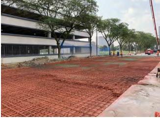
Fig. 8: Replacement roof slab ready to cast.
