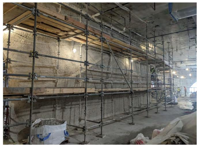
Fig. 8: After structural coat was set, shoring could be removed. This allowed for ample room to shoot the finish coat.
