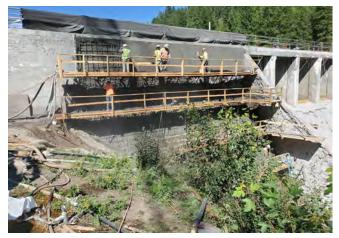
Fig. 10: Continuation of shotcrete placement at Moyie Dam, 2021.
