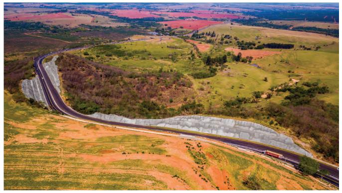
Fig. 1: Completed roadside slope connecting the towns of Marília and Assis in the state of São Paulo, Brazil.
