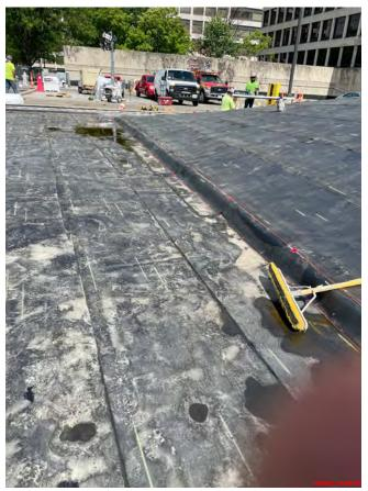
Fig. 5: Waterproofing membrane on exposed roof slab.
