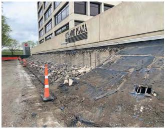
Fig. 4: Demolition of exterior slab.
