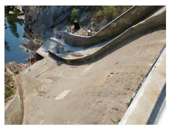
Fig. 4: Right spillway at Moyie Dam showing old shotcrete, 2021.
