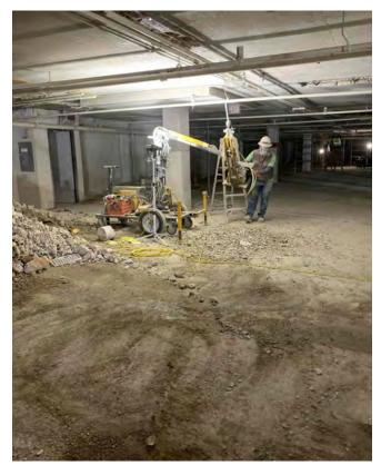
Fig. 10: Mechanically assisted chipping hammer for overhead demolition.
