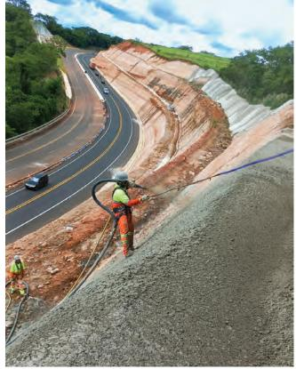
Fig. 7: Application of shotcrete using the rappelling technique.
