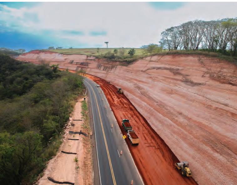
Fig. 3: Excavation and slope process for highway expansion.
