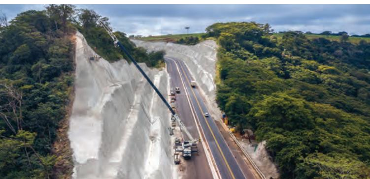
Fig. 5: Application of shotcrete from a man basket using a crane.
