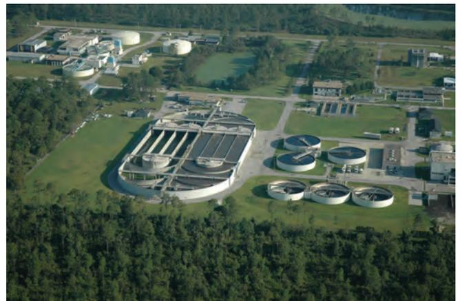
Fig. 4: Biological Nutrient Removal (BNR) tank, Daytona, FL.
