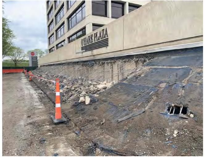
Fig. 4: Demolition of exterior slab.
