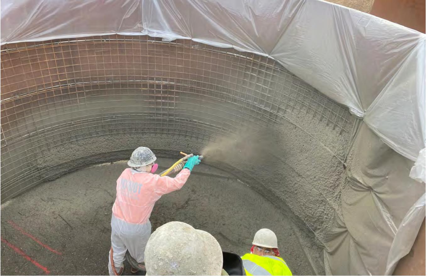
Fig. 3: Mock-up: Shotcrete placement.
