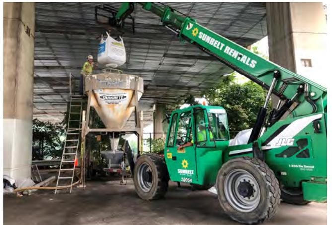
Fig. 7: Pre-packaged material, Quikrete Shotcrete MS, being loaded into a bulk hopper. The concrete repair mortar is then pre-dampened immediately prior to gunning and then water is added at the nozzle.
