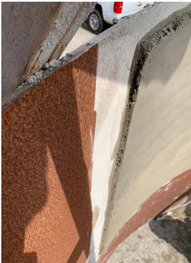
Fig. 2: Pipe after application of CML.
