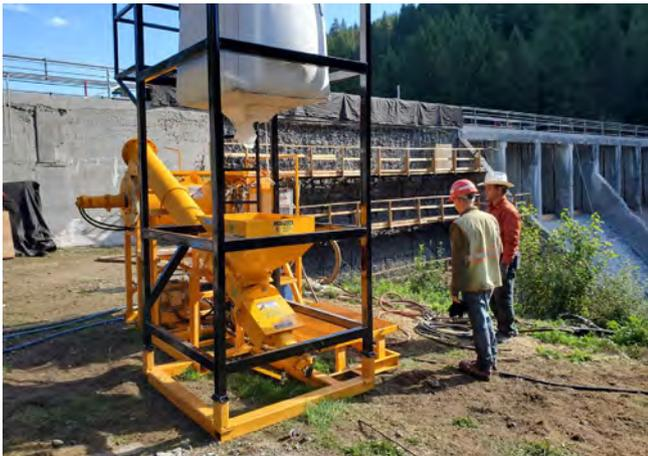
Fig. 7: Bulk bag hanger at Moyie Dam, 2021.
