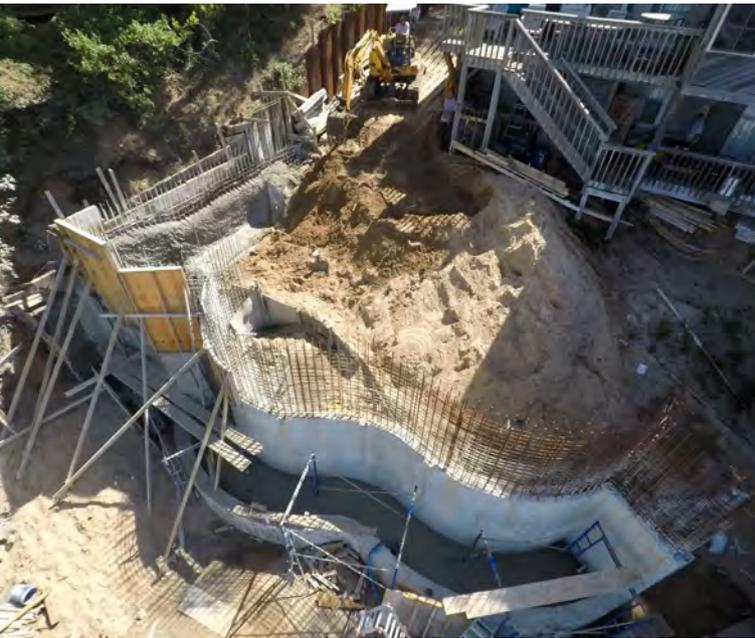
Fig. 7: Backfilling shotcreted walls.
