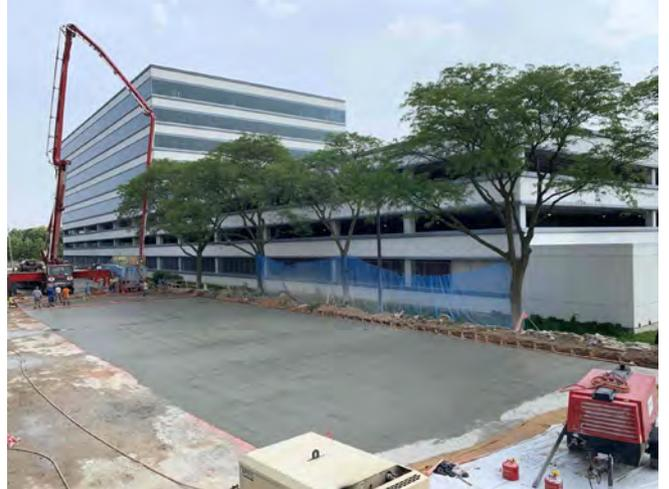
Fig. 9: Replacement roof slab.
