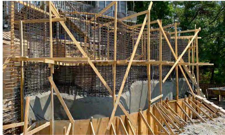
Fig. 5: View of bottom-up approach at ground level.
