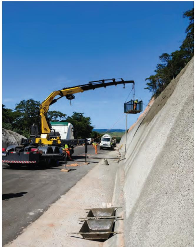
Fig. 9: Application of shotcrete using a truck-mounted crane.
