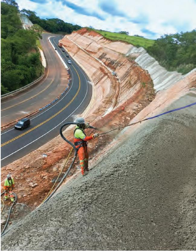
Fig. 7: Application of shotcrete using the rappelling technique.
