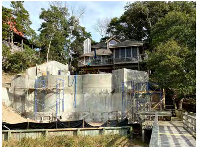
Fig. 10: Finished shotcrete view of the vanishing edge.
