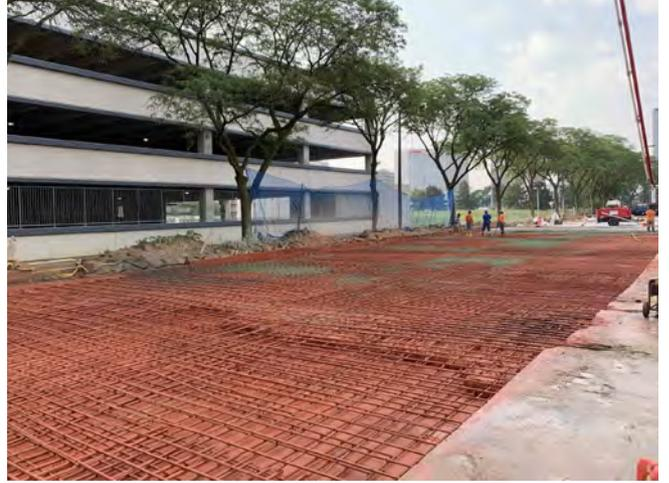
Fig. 8: Replacement roof slab ready to cast.
