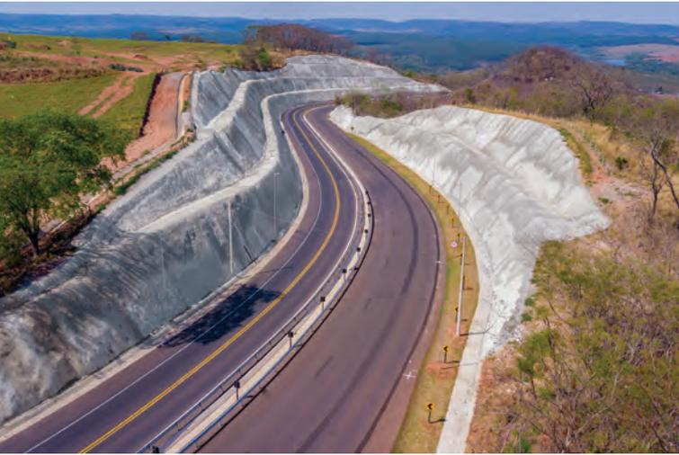
Fig. 10: Slope after shotcrete application.
