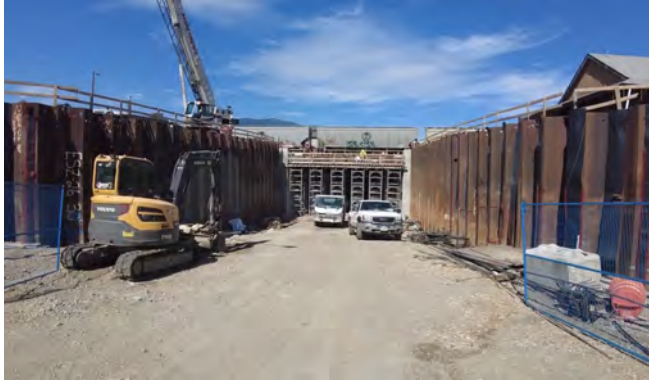
Fig. 2: Sheet piles used to stabilize the Ross Street Underpass.
