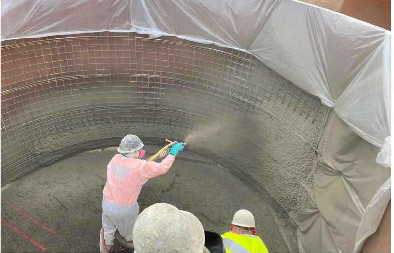
Fig. 3: Mock-up: Shotcrete placement.
