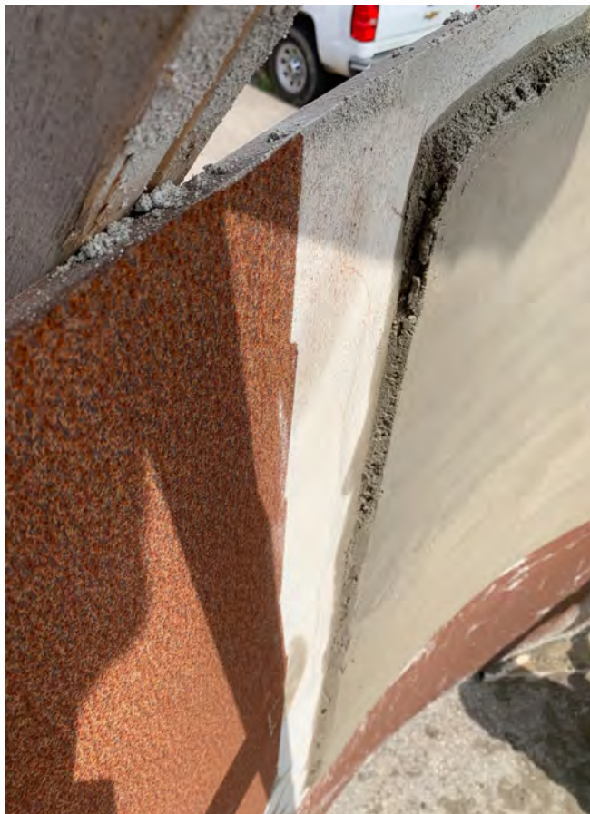
Fig. 2: Pipe after application of CML.
