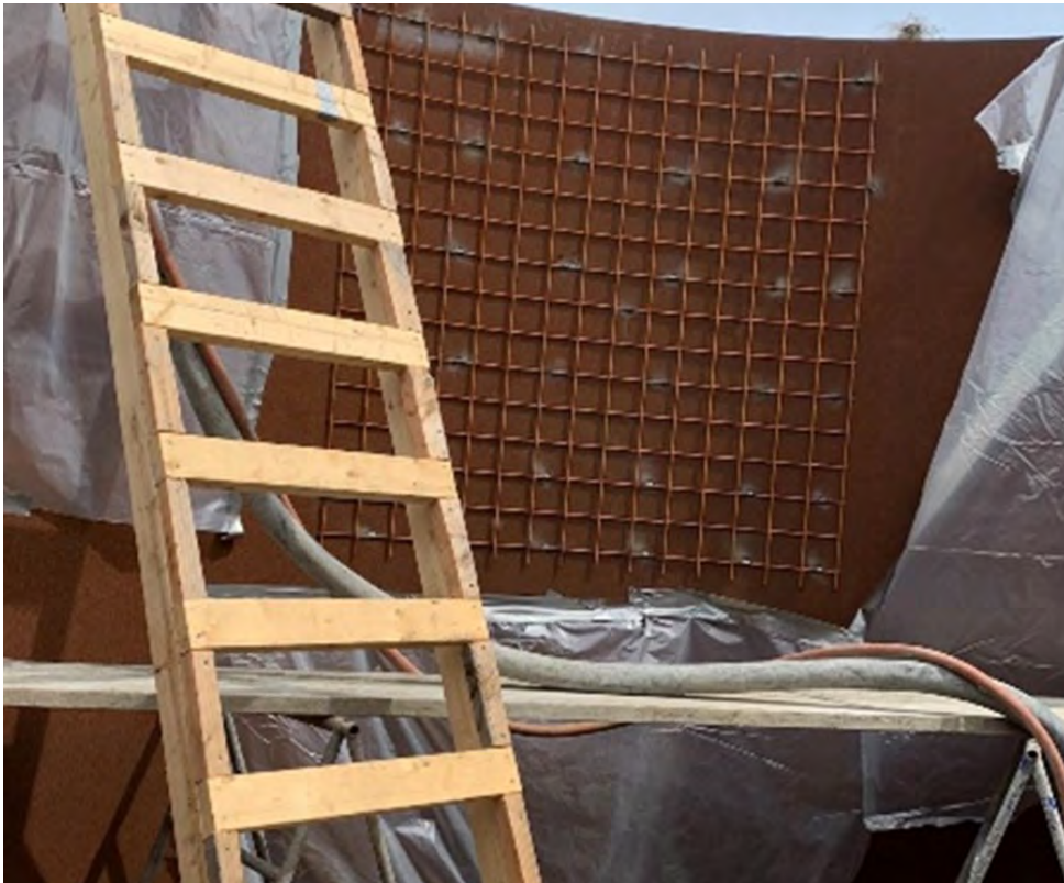
Fig. 1: Welded wire reinforcement tack welded to the steel pipe.
