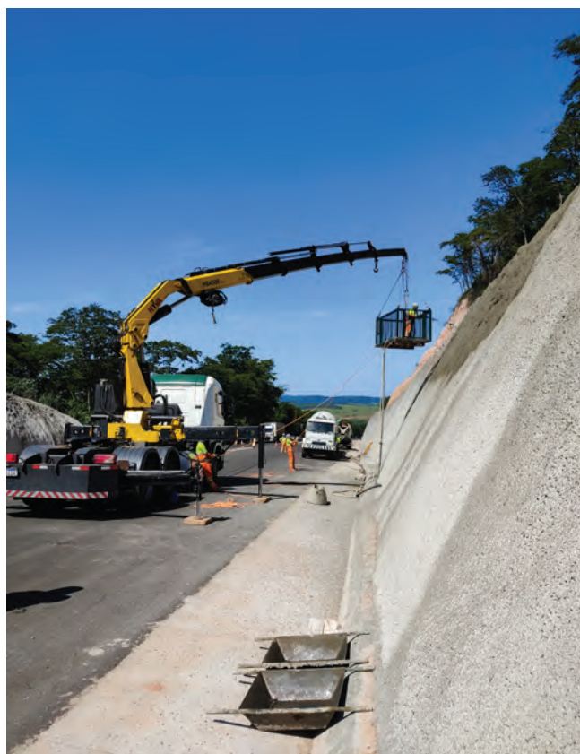
Fig. 9: Application of shotcrete using a truck-mounted crane.
