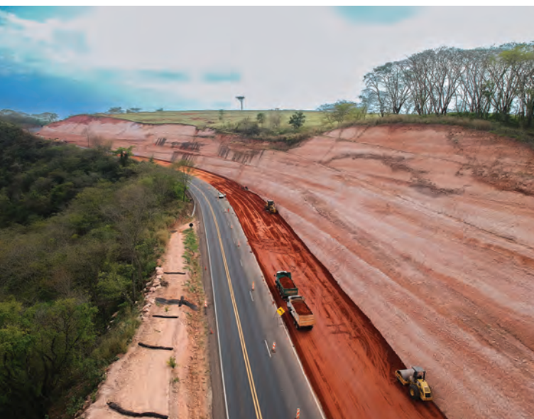
Fig. 3: Excavation and slope process for highway expansion.
