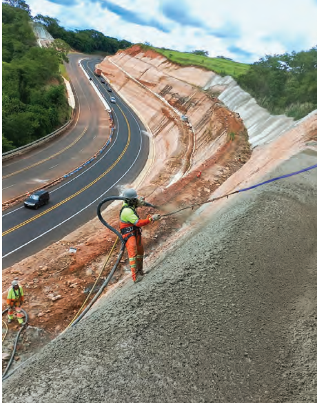
Fig. 7: Application of shotcrete using the rappelling technique.
