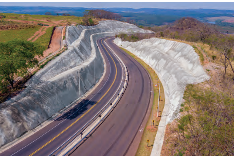
Fig. 10: Slope after shotcrete application.
