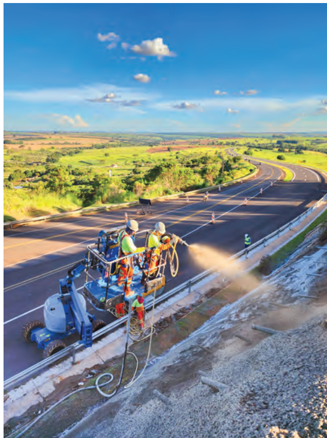
Fig. 8: Application of shotcrete using an articulating boom lift.
