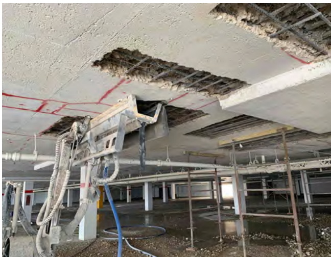
Fig. 2: Extensive deterioration inside the parking structure.
