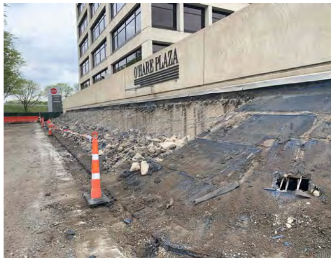
Fig. 4: Demolition of exterior slab.
