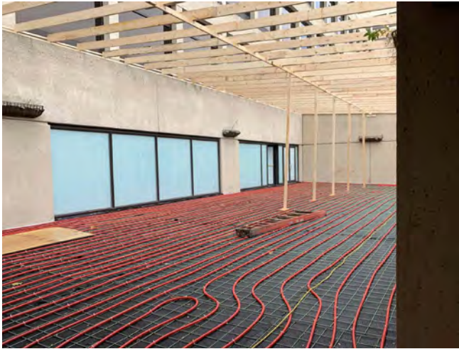
Fig. 11: Concrete slab with heating piping for melting ice and snow.
