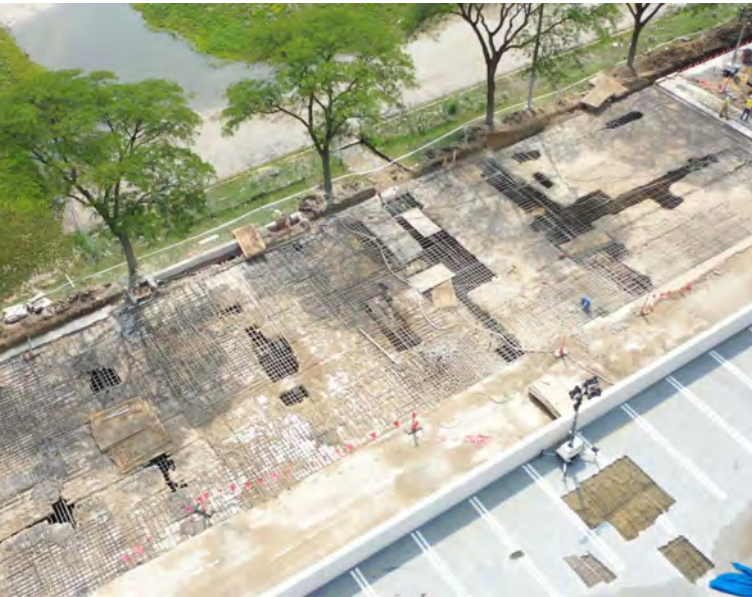
Fig. 6: Overview of roof slab with full depth repair areas apparent.
