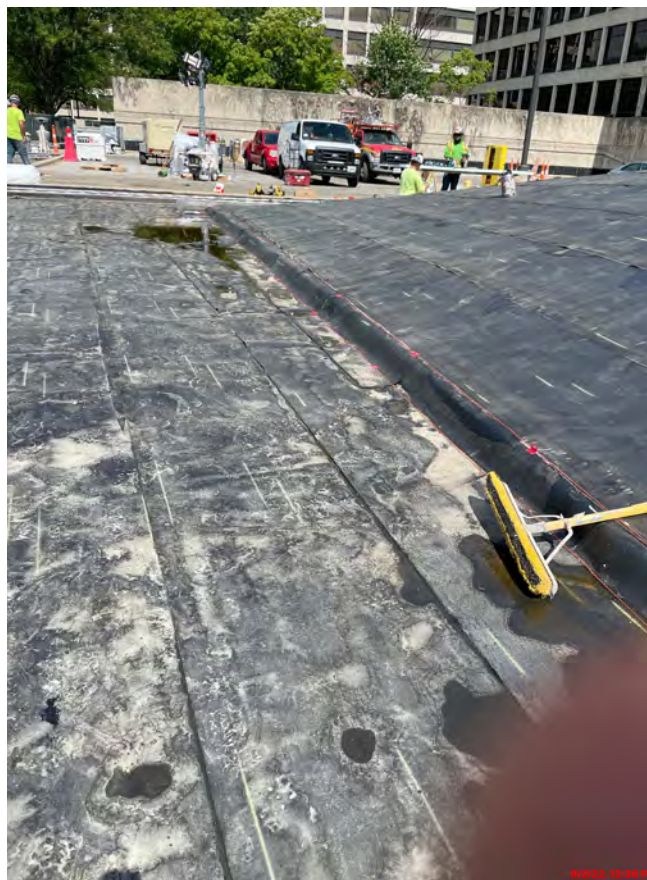
Fig. 5: Waterproofing membrane on exposed roof slab.
