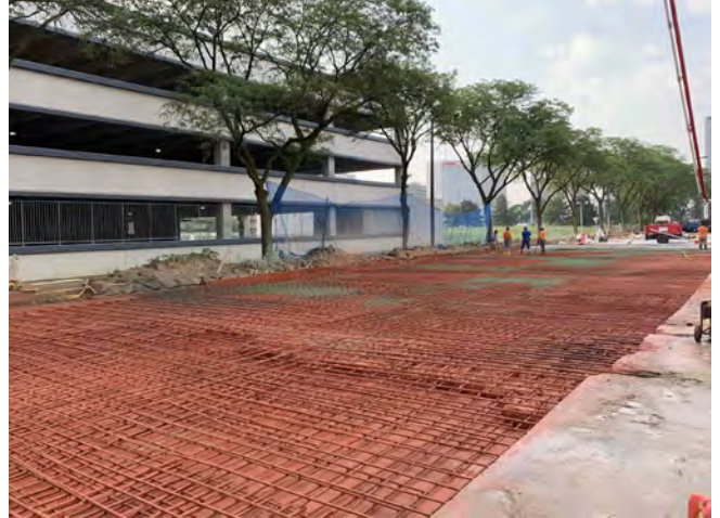
Fig. 8: Replacement roof slab ready to cast.
