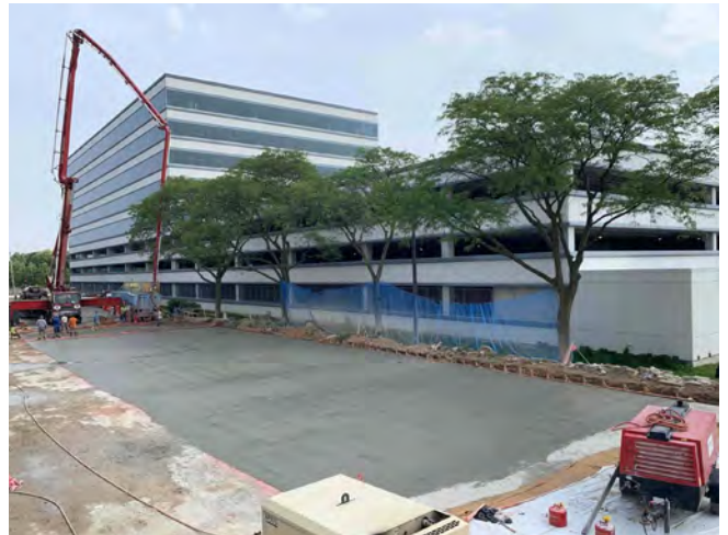
Fig. 9: Replacement roof slab.
