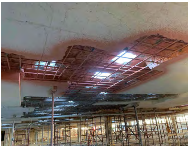
Fig. 3: Extensive deterioration inside the parking structure showing sunlight through the ceiling.
