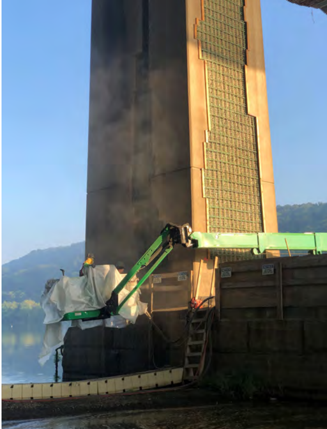
Fig. 10: Installing Shotcrete from a barge in the main channel of the Ohio River. Note the prepared area on the left face of the river pier.
