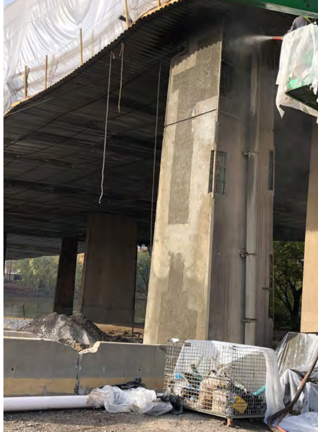
Fig. 6: Dry-mix shotcrete gunning of bridge pier to the right with finished sections to the left side of the pier.
