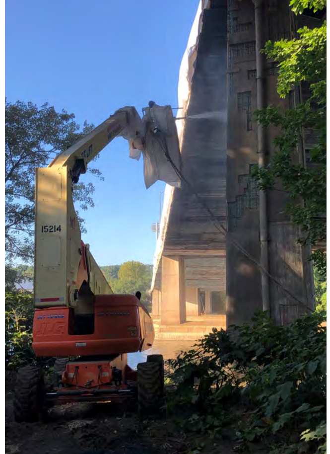
Fig. 9: Shotcrete being gunned in place on a riverbank pier. Dry-mix shotcrete works well with the stop and go nature of concrete repair applications.
