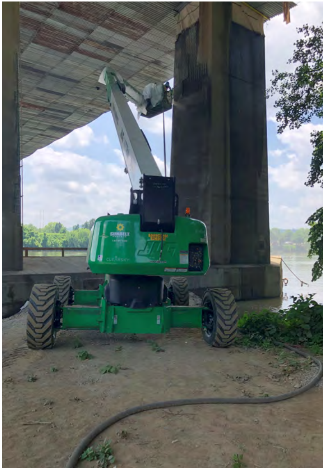
Fig. 2: Gunning a pier at the river's edge. When shooting from a man lift, each patch or area must be shot, cut down to grade and finished before moving on to the next.
