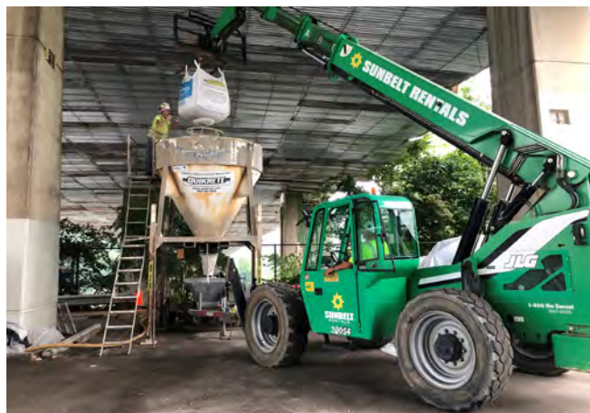
Fig. 7: Pre-packaged material, Quikrete Shotcrete MS, being loaded into a bulk hopper. The concrete repair mortar is then pre-dampened immediately prior to gunning and then water is added at the nozzle.
