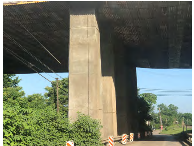
Fig. 13: Four gunned and completely finished piers in the Glenfield Borough section of the project.
