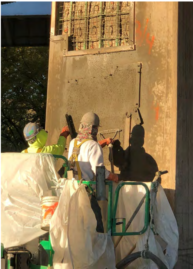
Fig. 11: The cutting-down and finishing work has to be done in a timely manner. Working out of man lifts necessitates a stop and go procedure.
