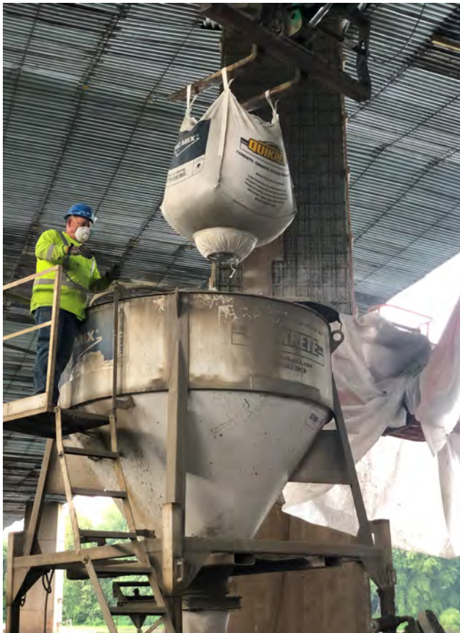
Fig. 8: Holding hopper being loaded with a 3,000 lb bag of pre-mixed material. The hopper holds 5 bulk bags of the Shotcrete repair mortar.
