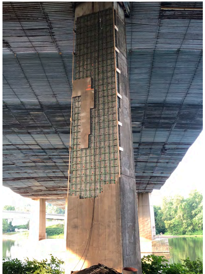
Fig. 4: A pier is prepped and ready for gunning.
