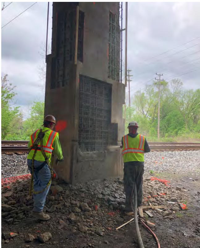
Fig. 5: Shooting a pier on an approach span on the south end of the Neville Island Bridge.
