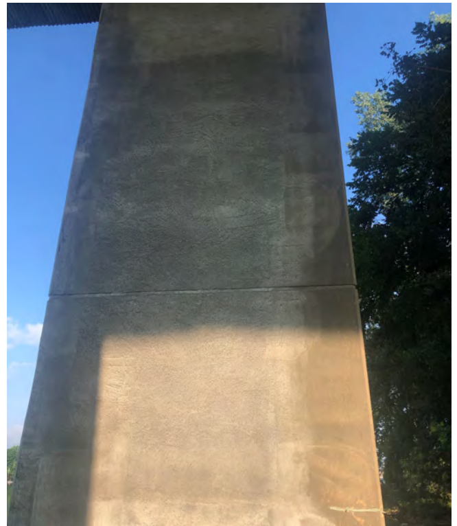
Fig. 12: A close-up picture of a bridge pier with the newly installed shotcrete adjacent to the existing concrete.
