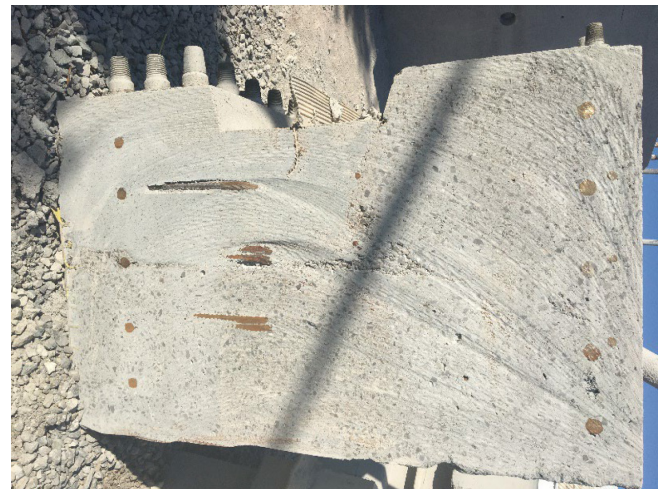
Fig. 9: Another example of a wire saw cut section of mockup showing excellent quality of shotcrete at the transition between the shotcrete and the self-consolidating poured concrete
