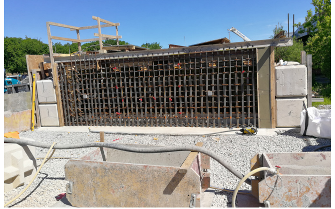
Fig. 7: Full-scale 1.3 m thick station wall mock-up
