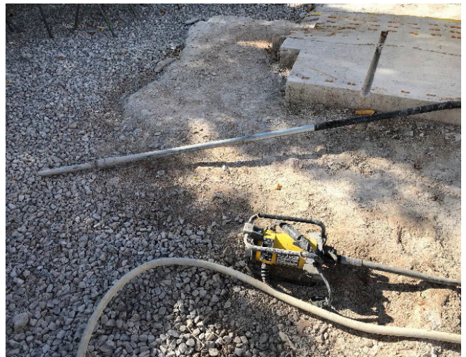
Fig. 5: A long 40 mm (1.5 in.) diameter stiff rod vibrator provided the placed shotcrete with supplementary consolidation. Credit: Jimmy Wang.
