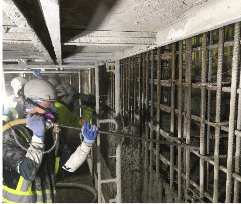
Fig. 4: Compressed air blow pipe working in tandem with nozzleman during bench shooting.
