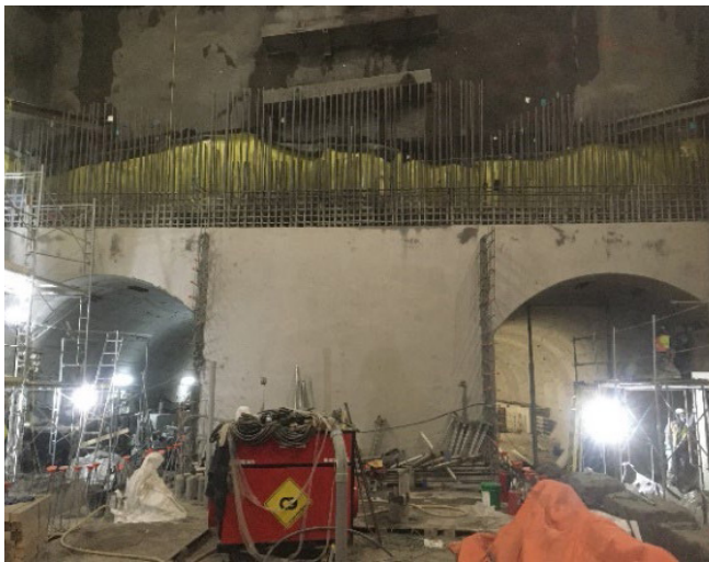
Fig. 2: Shotcrete wall construction at tunnel openings
