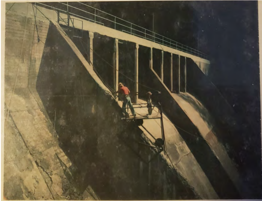
Fig. 1: Prep Training at Moyie Dam, 1981.
