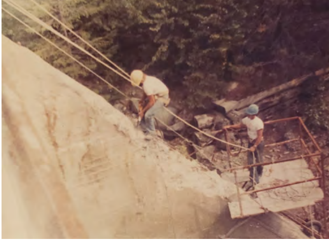
Fig. 2: Prep at Moyie Dam, 1981.
