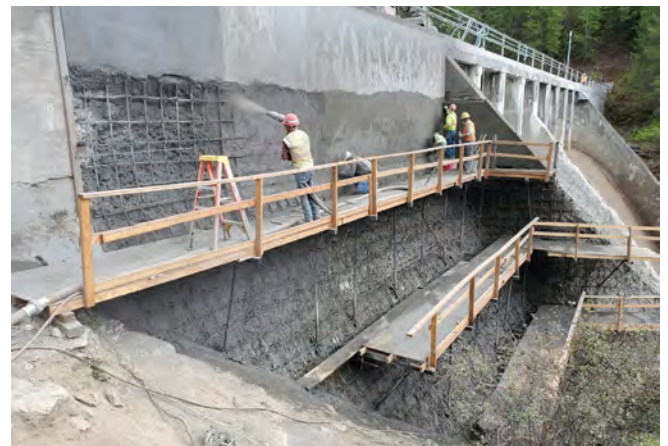
Fig. 9: Nozzlemen placing and finishing new shotcrete at Moyie Dam, 2021.
