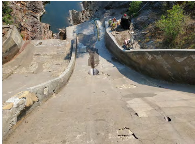
Fig. 5: Left spillway at Moyie Dam showing old shotcrete, 2021.
