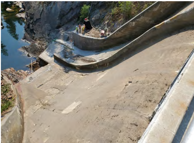
Fig. 4: Right spillway at Moyie Dam showing old shotcrete, 2021.
