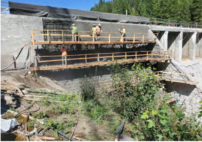
Fig. 10: Continuation of shotcrete placement at Moyie Dam, 2021.
