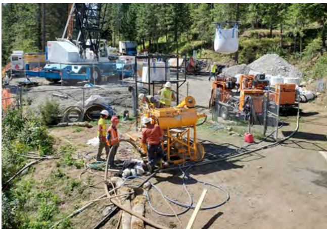
Fig. 8: View of equipment staging at Moyie Dam, 2021.
