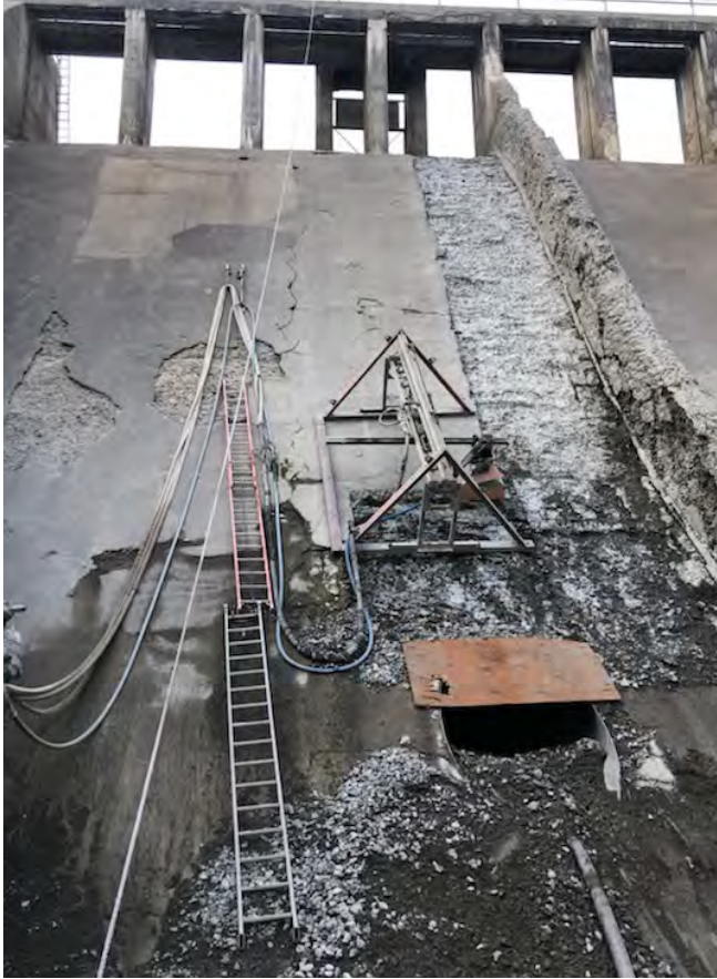
Fig. 6: Hydro demolition at Moyie Dam, 2021.
