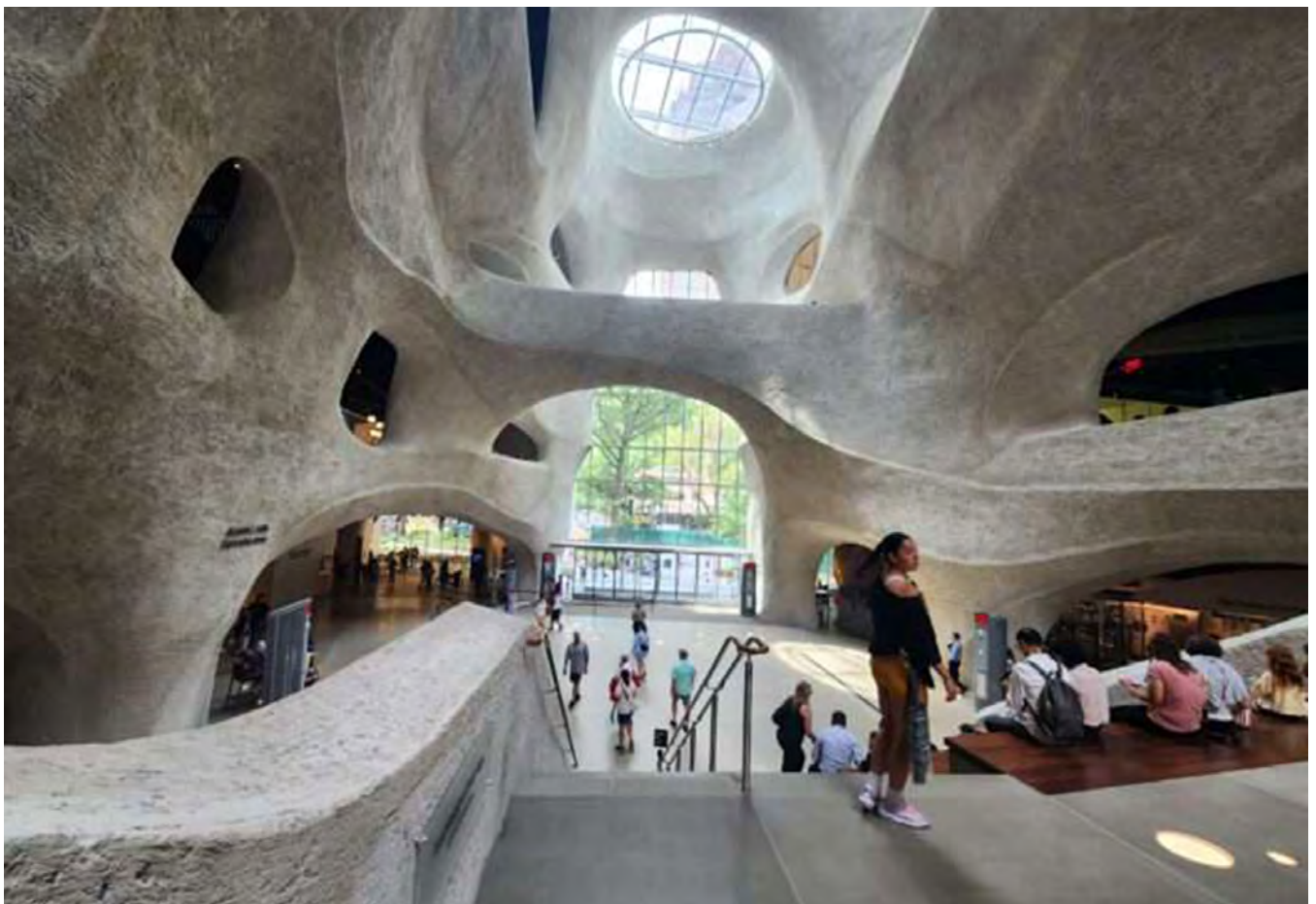
Fig. 1: COST of Wisconsin used specialized shotcrete and rebar techniques to construct the interior and exterior walls of the Gilder Center at AMNH. All photos are courtesy of COST of Wisconsin.
