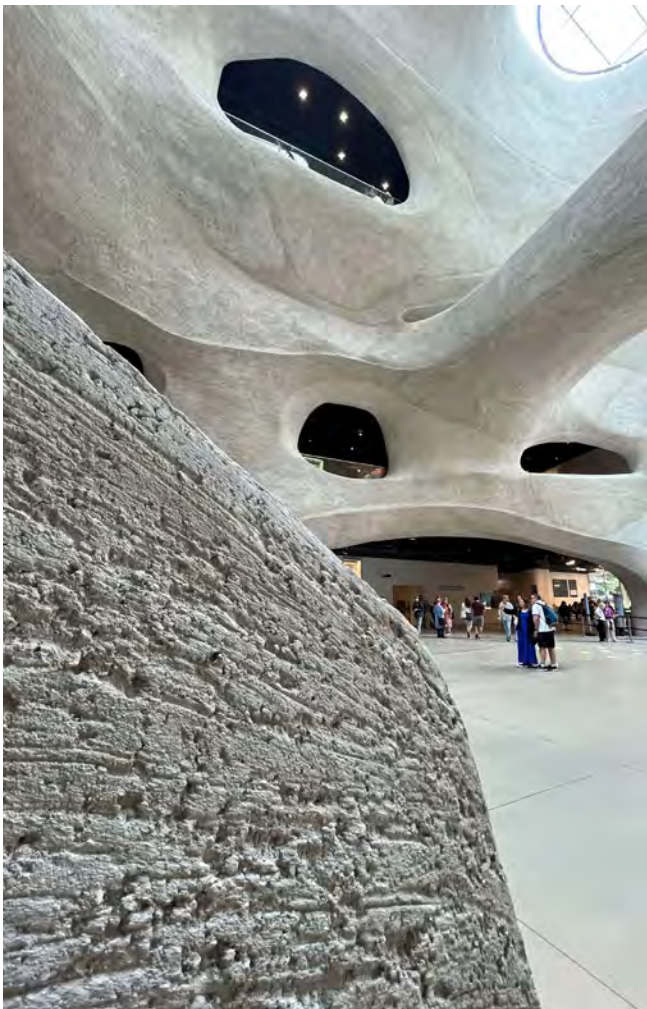
Fig. 12: The walls have a unique texture and pigmentation. The white cement was sourced locally from Lehigh, New York.
