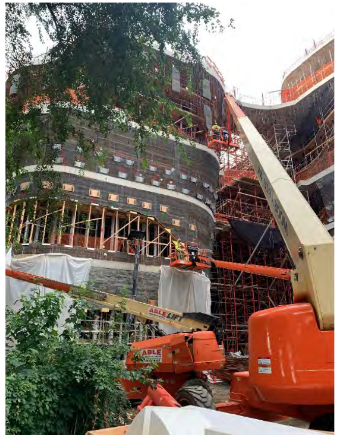
Fig. 10: Exterior work - 5 crews working in separate locations.
