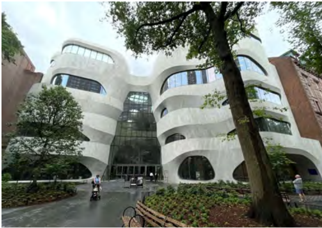
Fig. 11: Gilder Center—completed exterior.
