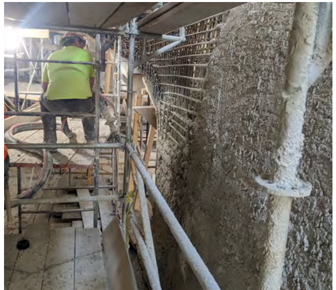
Fig. 7: Average workspace when shooting the structural layer of shotcrete.
