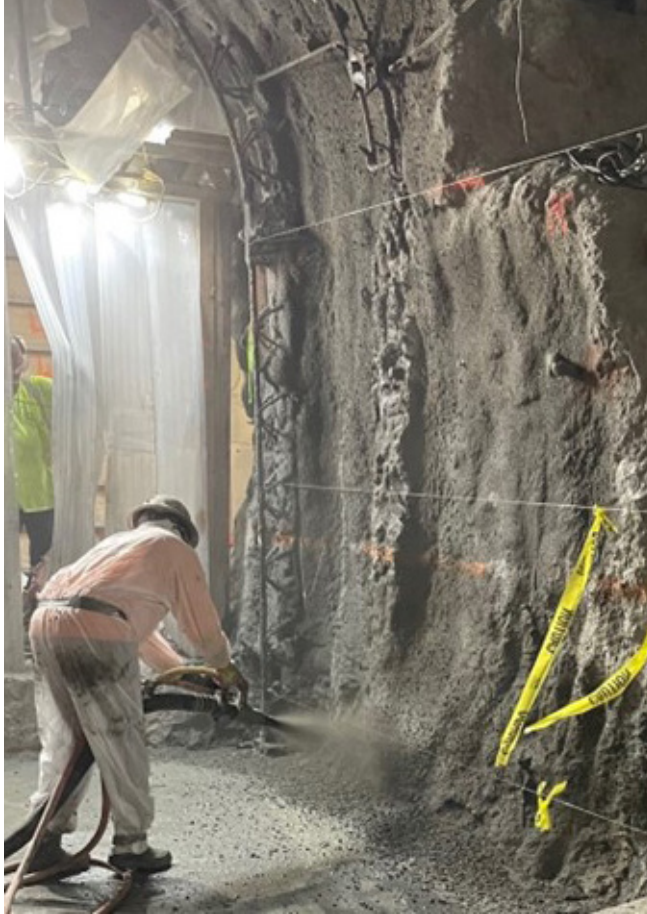
Fig. 5: Smoothing coat being applied
