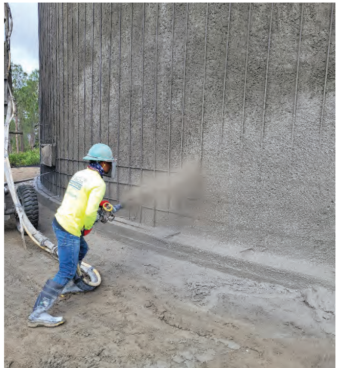
Fig. 8: CROM ACI-Certified Nozzleman shooting shotcrete.
