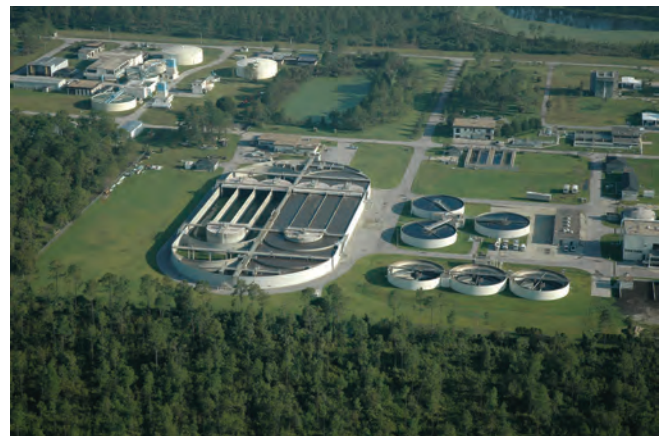
Fig. 4: Biological Nutrient Removal (BNR) tank, Daytona, FL.
