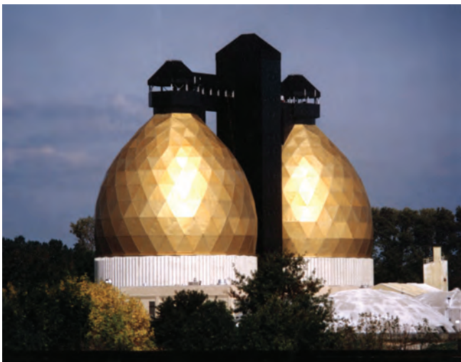
Fig. 1: Egg-Shaped Digester Tanks, Baltimore, MD.
