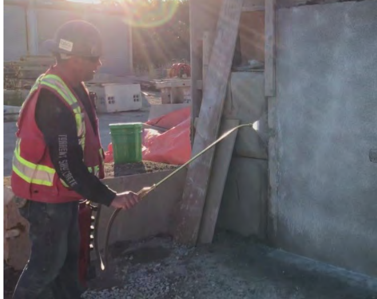
Fig. 18: Finished mock-up was cured using a spray on applied curing compound. Photo Credit: Jimmy Wang.
