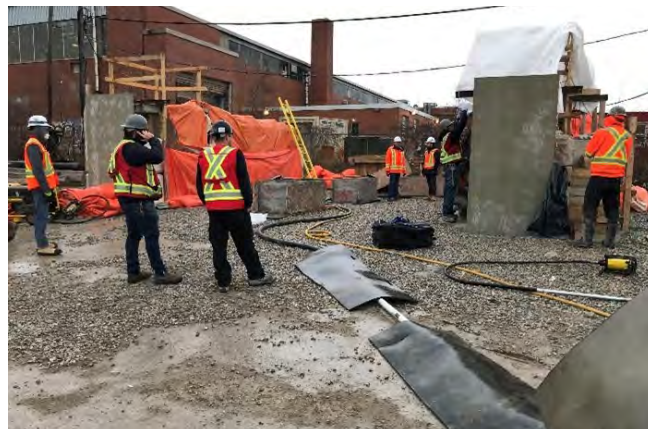
Fig. 4: Steel slickline and rubber hose which fed shotcrete to the mock-up. Credit: Jimmy Wang.
