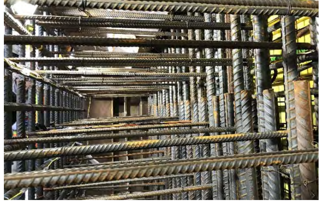
Fig. 9: Inside mock-up showing spliced 25M vertical reinforcing (inner wall face), spliced 3-35M vertical reinforcing (outer wall face), 15M holder bars and plastic waterstop.
