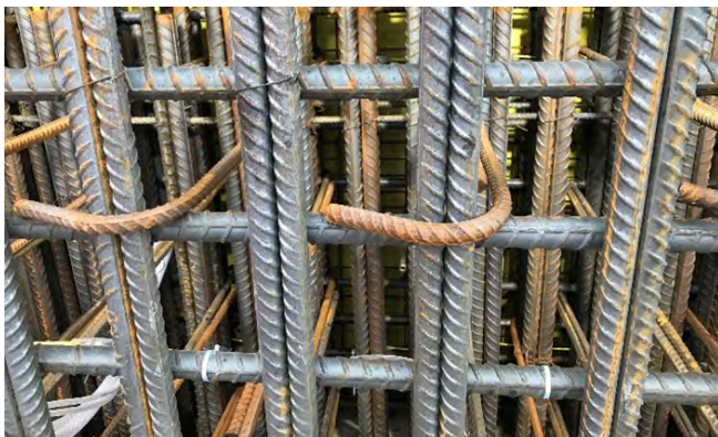
Fig. 8: Mock-up was heavily reinforced with 4 layers of heavy rebar, including 3 layers of closely spaced 35M (#9) rebar at the back of the work adjacent to a water proofing membrane. Photo Credit: Jimmy Wang
