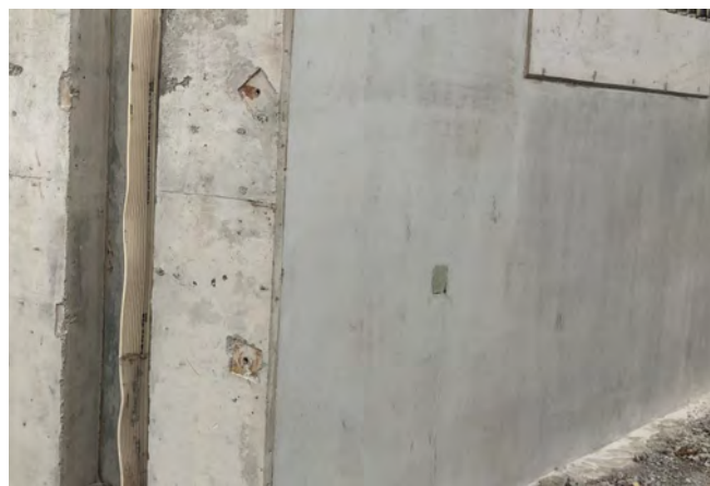
Fig. 19: Finished mock-up following stripping of the formwork after curing in air for 10-days.
