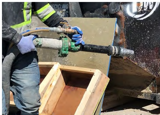
Fig. 5: Nozzle assembly utilizing a unique pipe extension between the rubber nozzle tip and the nozzle air ring compressed air valve. Rubber nozzle tip is wrapped tight with grey duct tape. Credit Jimmy Wang.
