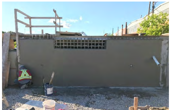
Fig. 16: Final finishing of mock-up. Photo Credit: Jimmy Wang.
