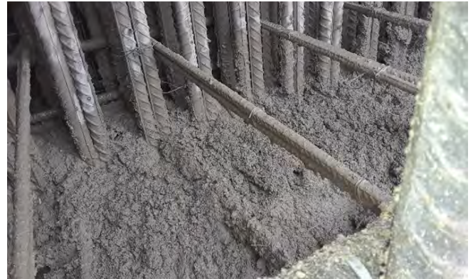
Fig. 14: Following use of stiff rod vibrator, shotcrete was being well consolidated and wrapping around the three outer 35M reinforcing steel bars. Photo Credit: Leonard Crasta.
