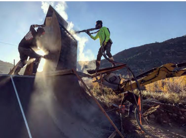
Fig. 9: Sunrise Silhouette—In the early morning light, Mark Bradford casts a shadow while he skillfully shoots a spray of concrete. Placement and consolidation are crucial. Project: Lake Crowley Skatepark, Lake Crowley, CA.
