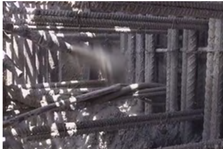
Fig. 11: Nozzleman inserting entire nozzle tip and extension between square openings in the front mat of reinforcing steel. Shotcrete stream impacting three layers of vertical reinforcing steel and water proofing membrane at a high impacting velocity. Blow pipe being used to continuously clean the back reinforcing steel in front of the area about to be shot.
