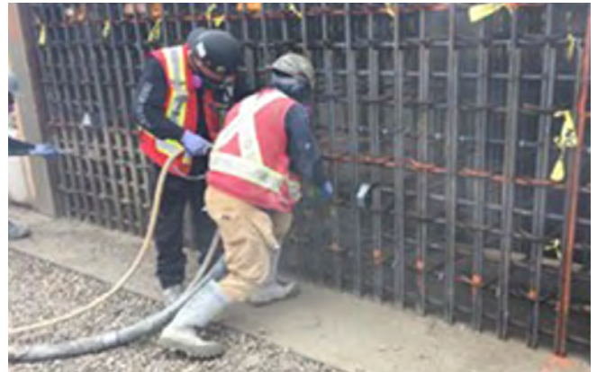
Fig. 10: Nozzleman bench shooting mock-up with blow pipe operator working in tandem with the nozzleman.
