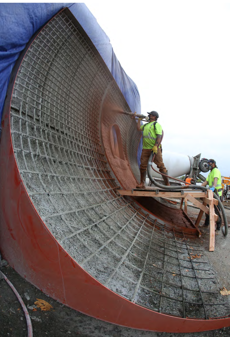
Fig. 3: A Cresting Vert Wall—SR Crew Lead and ACI-certified Nozzleman, Kelly Malobovich, sprays colored shotcrete onto an over-vert, free-standing concrete wall in La Puente, CA (2020). Project: Central Park Skatepark. Photographer: @Mikendo.
