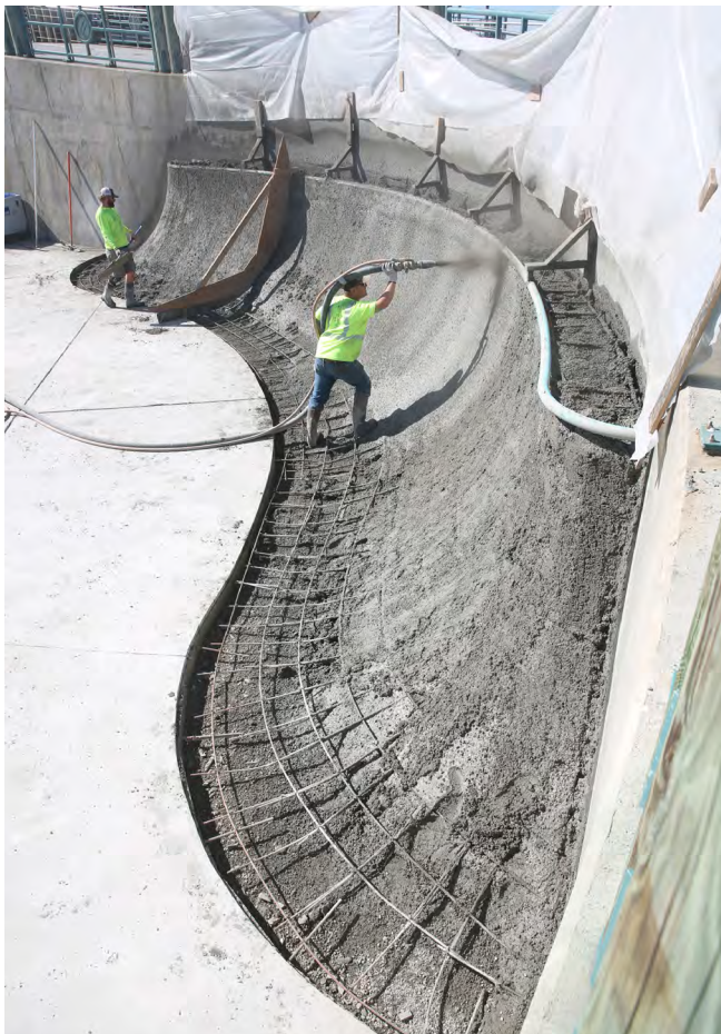
Fig. 7: Working the Wall—SR Crew Lead and ACI-certified Nozzleman Kelly Malobovich applies concrete to a crucial consolidation area beneath the steel coping of a new skate spot feature at the Redondo Beach Pier in California (2023). Project: Redondo Beach Pier Skatespot. Photographer: @Mikendo.
