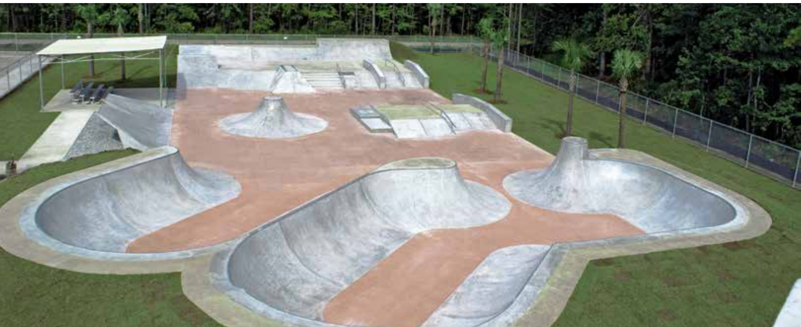
No flat surfaces here—shotcrete is a natural choice for this project
