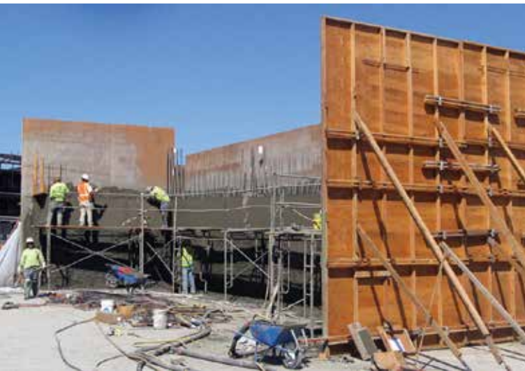
Shotcrete sprayed in place against one-sided forms saves 50% of the forming required in cast-in-place installations
