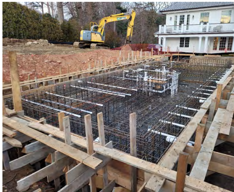
Fig. 2: Complex reinforcing with integral spa and embedded piping. Not a simple design or construction (Photo courtesy of Drakeley Pools).
