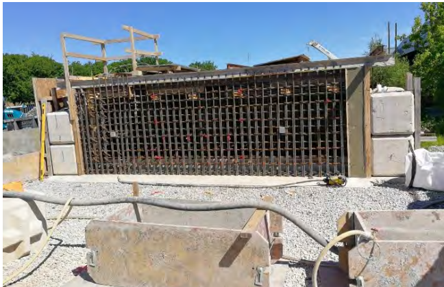
Fig. 7: Full scale 1.3 m (51 in.) thick mockup. Photo Credit: Robert Mattes
