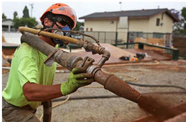
Fig. 8: ACI-certified Nozzleman, and article co-author, Mark Bradford, in his element in Hawaiian Gardens, CA. Project: Clarkdale Skatepark. Photographer: @Mikendo.
