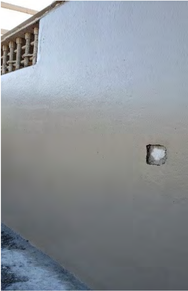
Fig. 17: Close up view of the finished mock-up. Photo Credit: Mitchell Matais.
