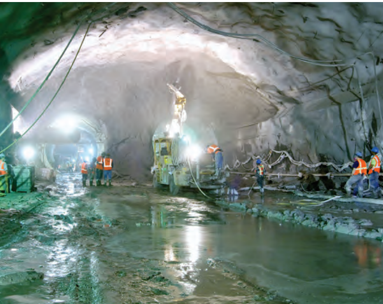
Fibercon steel reinforcing fibers used in East Side Access Tunnel, NYC
