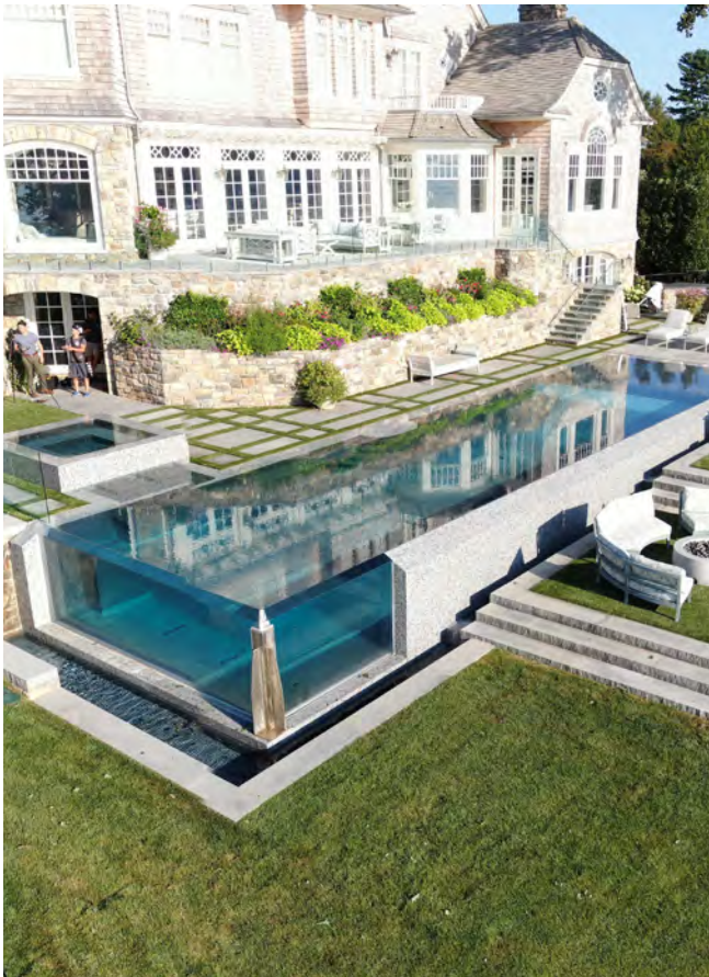
Fig. 1: Partially buried, embedded window, infinity edge residential pool. Not just a basic backyard swimming hole (Photo courtesy of Drakeley Pools).
