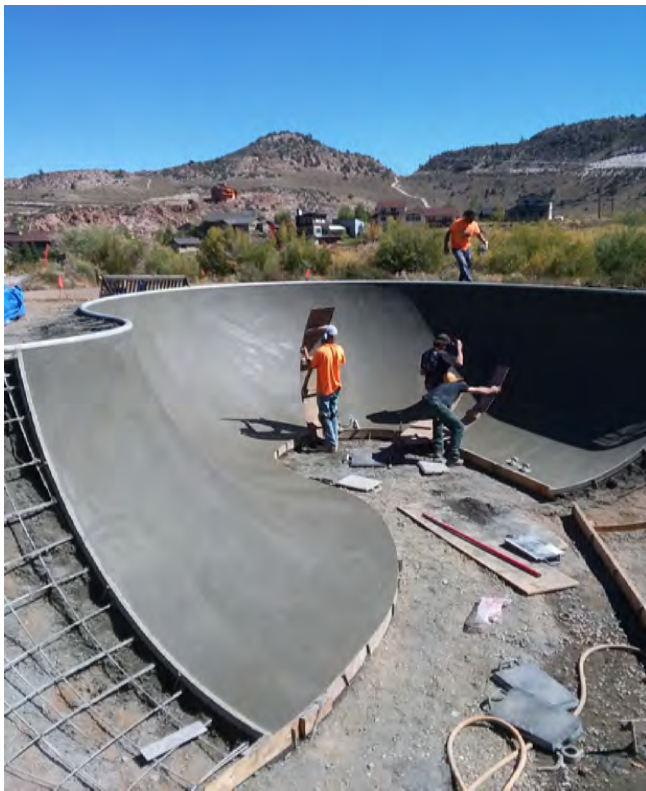
Fig. 5: Velvety Fresh —The sweeping shotcrete curves of a clover bowl in Crowley Lake, CA begin to take shape (2017). Pictured: Spohn Ranch Build Team. Project: Lake Crowley Skatepark. Photographer: Mark Bradford.
