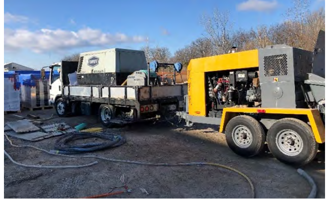
Fig. 3: 375CFM Air Compressor and Putzmeister TK60HP Shotcrete Pump.
