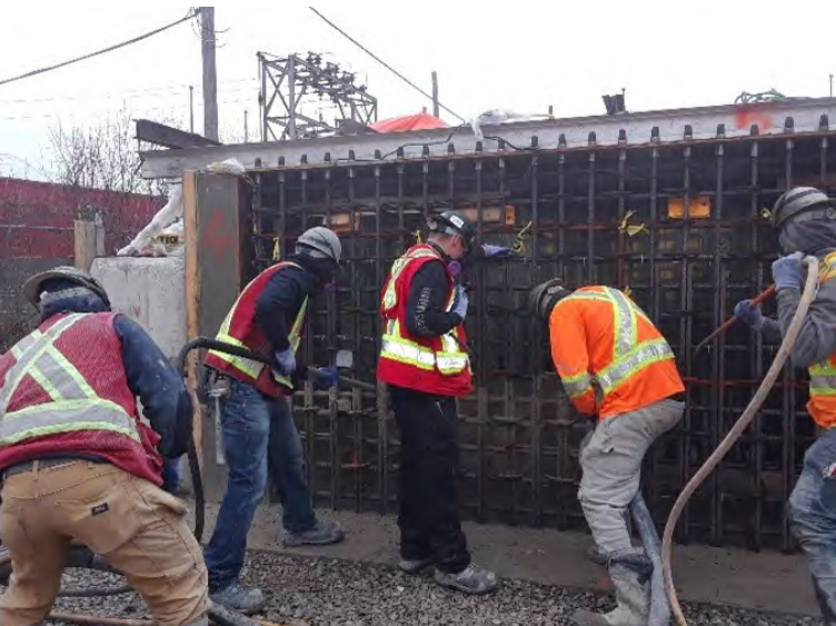
Fig. 12: An operator of a stiff rod vibrator would start behind the nozzleman inserting the vibrator to the back of the work to “lay down the bench” and provide supplementary consolidation of the shotcrete around the back-reinforcing steel. Photo Credit: Leonard Crasta.
