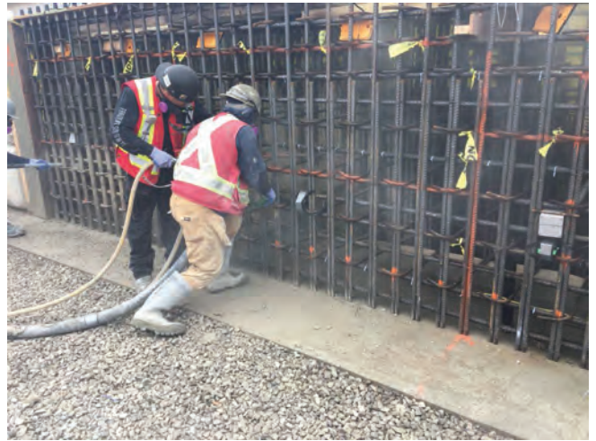
Fig. 7: Nozzleman and blow pipe operator shooting a congested test panel; framed using the Rule of Thirds.
