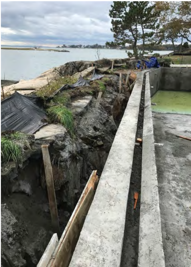
Fig. 3: Executing the precise edge detail required zero tolerance construction and dogged adherence to all applicable workmanship standards.
