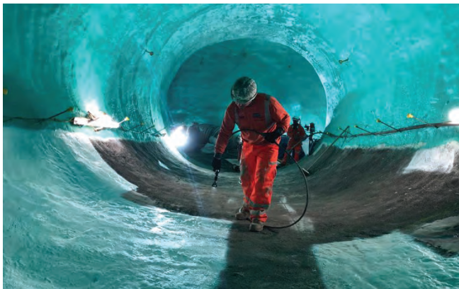
Fig. 1: Waterproofing System Application
