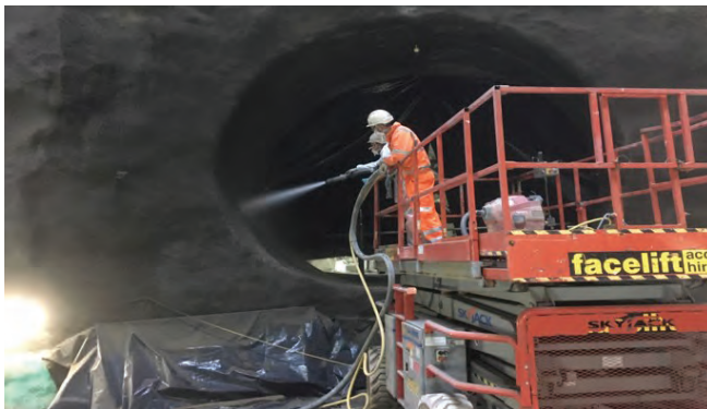
Fig. 6: Nozzlemen at a tunnel entrance
