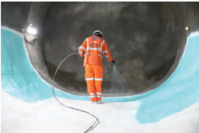
Fig. 10: Nozzleman applying waterproofing layer
