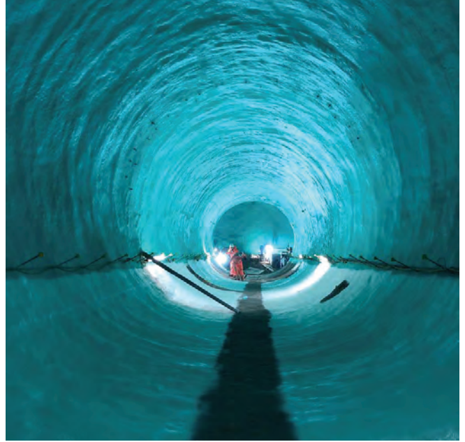
Fig. 11: Full tunnel view with waterproofing
