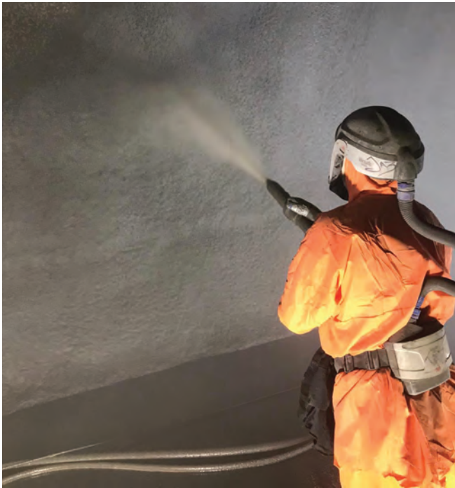
Fig. 8: Nozzleman applying Mapegrout Gunite FSD
