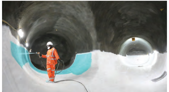
Fig. 2: Waterproofing System Application
