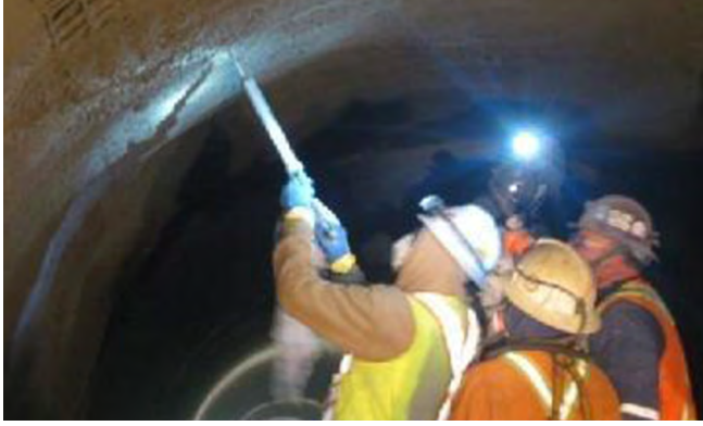
Fig. 7: In-place set time test
