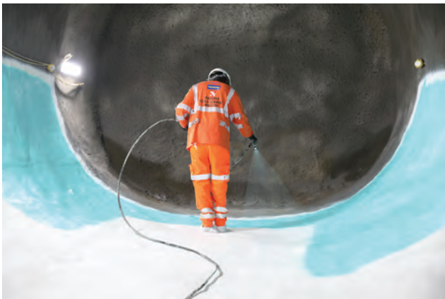
Fig. 10: Nozzleman applying waterproofing layer
