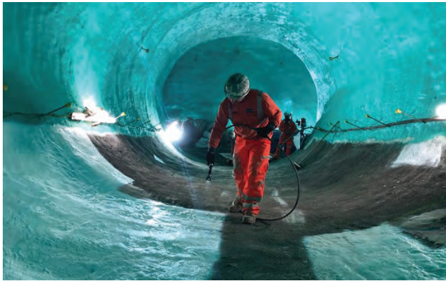
Fig. 1: Waterproofing System Application
