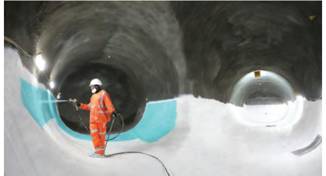
Fig. 2: Waterproofing System Application
