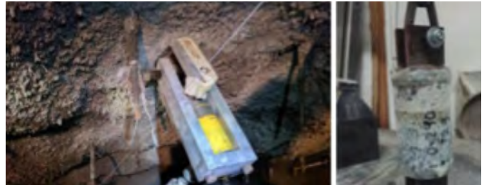
Fig. 10: In-place shotcrete bond strength test and laboratory shotcrete bond strength test
