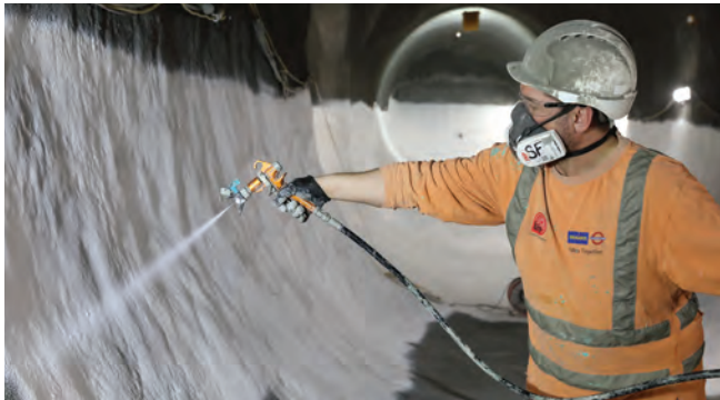
Fig. 5: Mapelastac TU System Application
