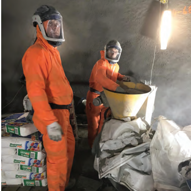
Fig. 4: Preparation of Mapegrout Gunite FSD
