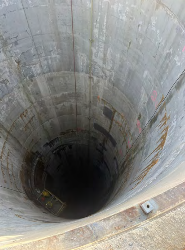
Fig. 7: Completed shaft repairs.
