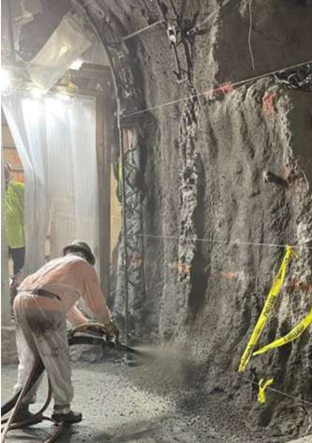
Fig. 5: Smoothing coat being applied
