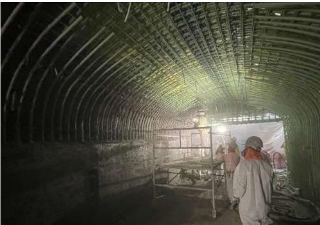
Fig. 6: Structural placement underway
