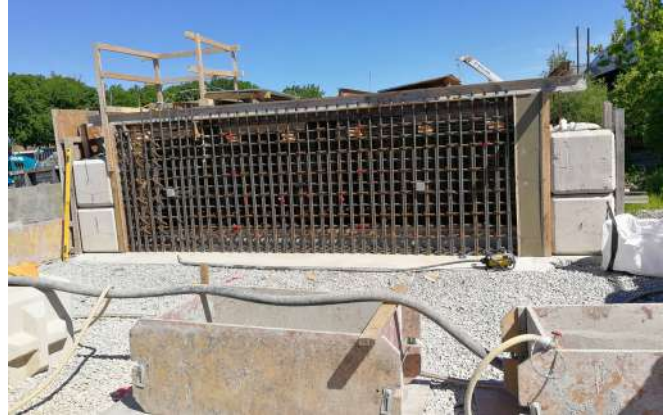
Fig. 7: Full-scale 1.3 m thick station wall mock-up
