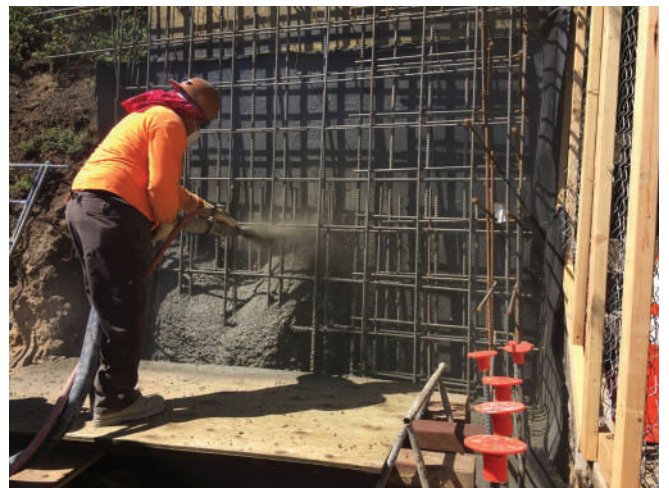
Wetsuit® 2-Part spray applied membrane behind shotcrete
