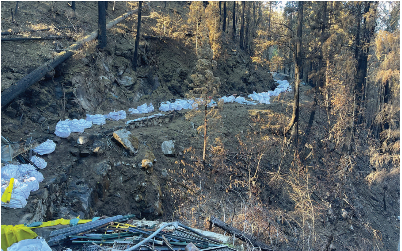
Fig. 1: Before shotcreting of the flume
