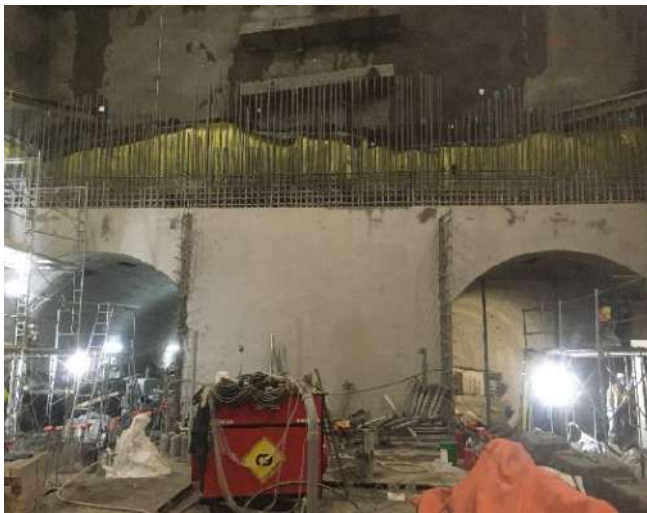
Fig. 2: Shotcrete wall construction at tunnel openings
