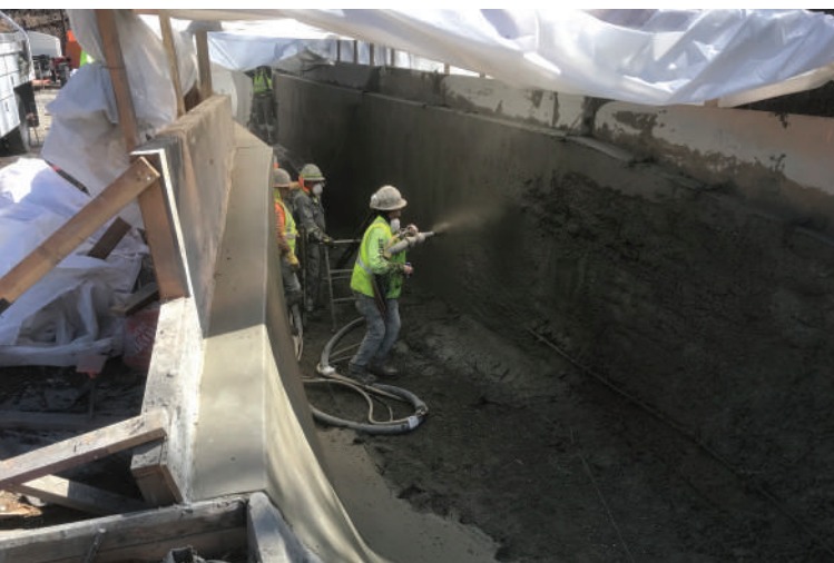
Fig. 6: Shotcrete walls
