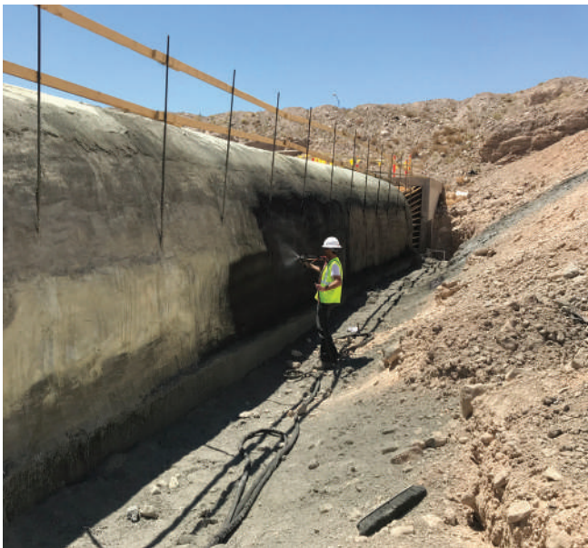
Wetsuit® 2-Part spray applied membrane over shotcrete
