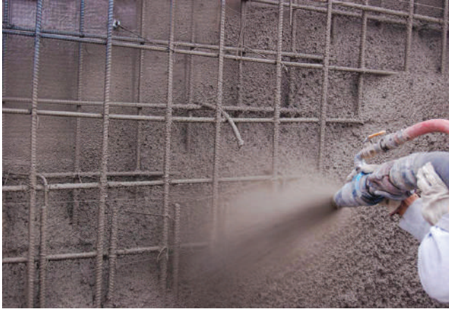
Shotcrete over Wetsuit® 2-Part spray applied membrane
