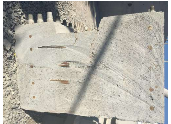
Fig. 9: Another example of a wire saw cut section of mockup showing excellent quality of shotcrete at the transition between the shotcrete and the self-consolidating poured concrete
