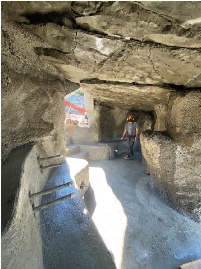
Fig. 2. Grotto roof and suspended slab finish.
