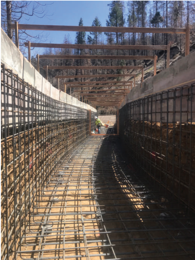
Fig. 3: Canal before shotcrete
