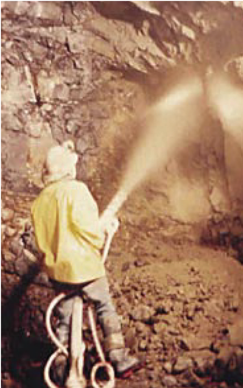
Tunnel construction provided a proving ground for new materials and equipment
