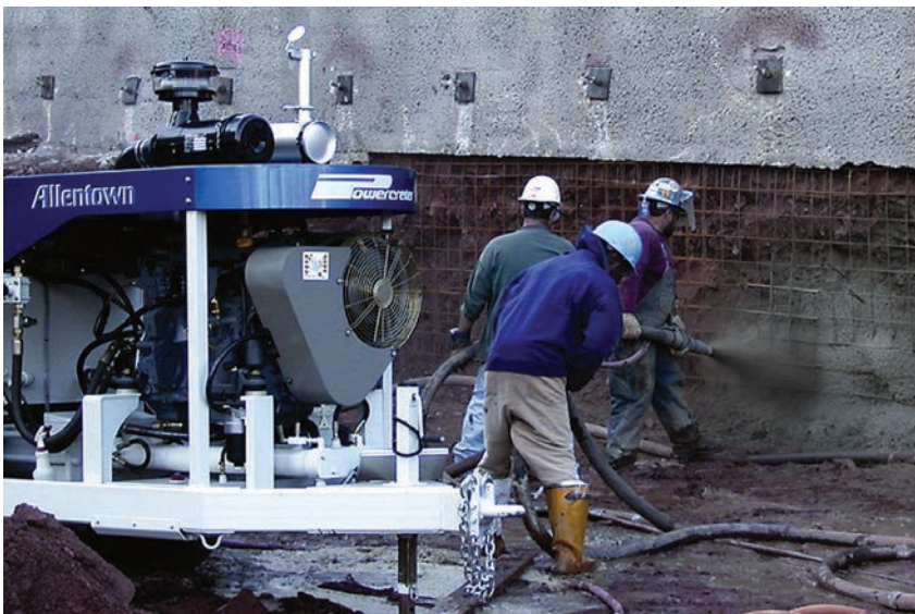
Fig. 3: Pump, nozzlemaster, and hose tenders
