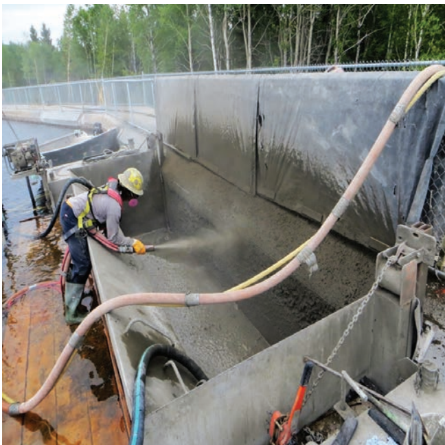
Fig. 1: Remote dam repair using dry-mix shotcrete and a cofferdam 1
