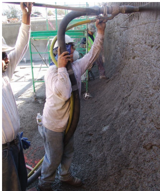
Fig. 1: Nozzlemaster with his air lance man and hose tender
