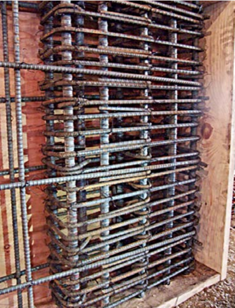
Fig. 3a & 3b: Different reinforcement configurations require different material consistencies.
