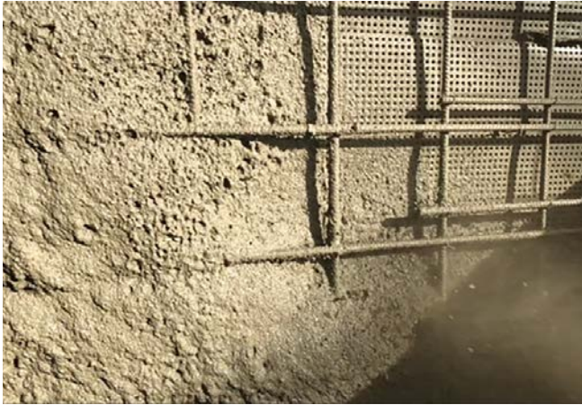
Fig. 7. The ideal slump allows incoming aggregates to deeply embed within the puddle rather than remaining on the surface.
