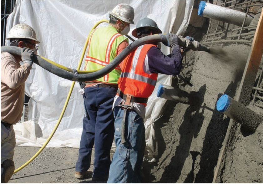
Fig. 1: Nozzlemaster with his air lance man and hose tender
