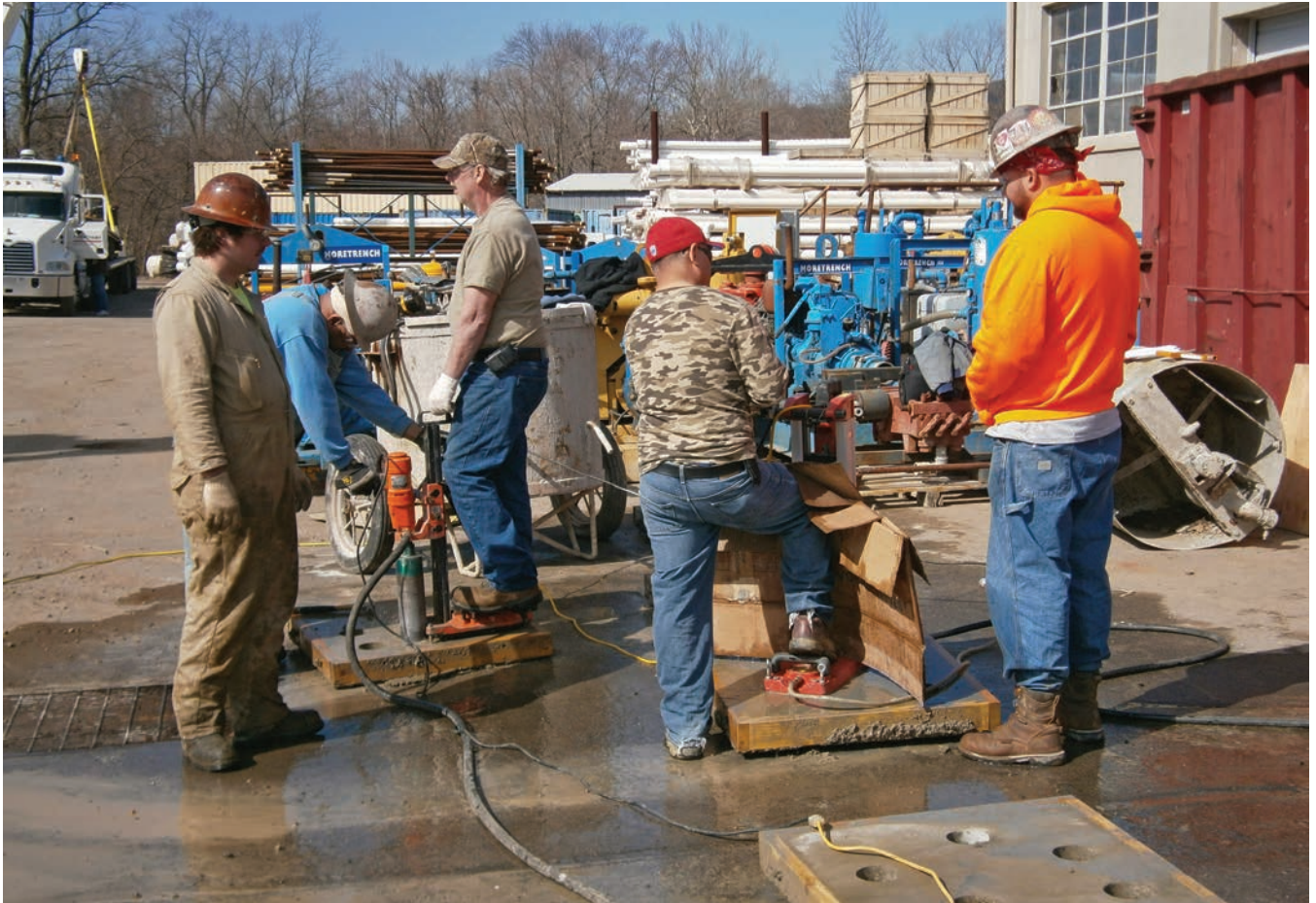
More than one core drilling rig with crews who have experience in the operation
