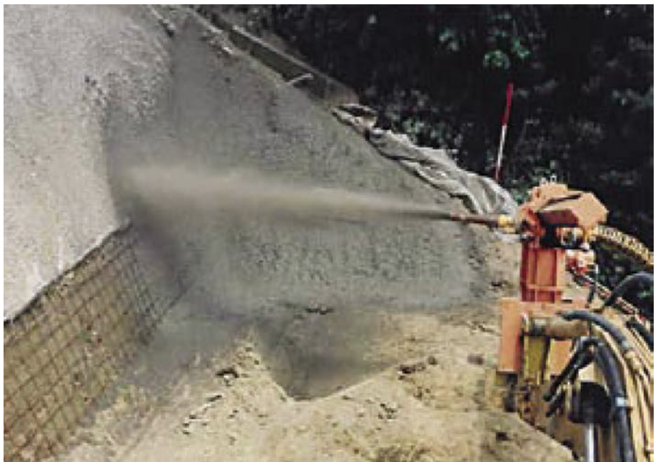
Automated wet-mix shotcrete for a geotech application
