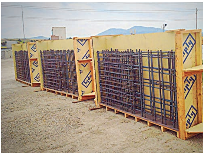
Fig. 1: Mockup panels with congested reinforcement patterns may require alternative methods to attain adequate consolidation
