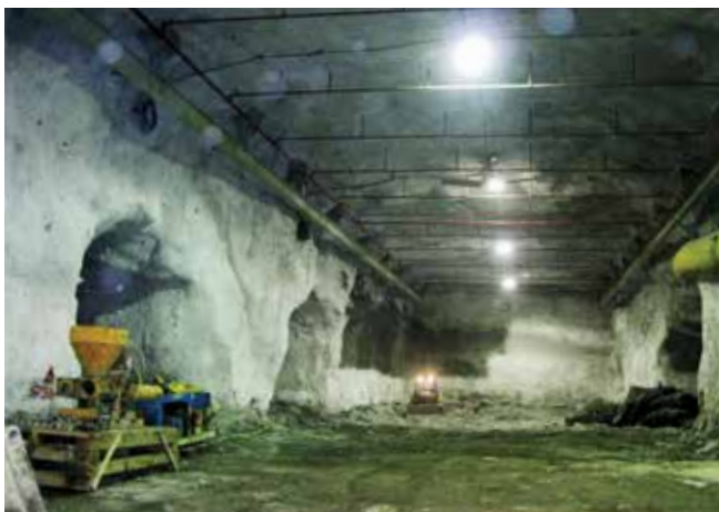
Fig. 9: Large underground opening for workshop in mine in Sudbury, ON, Canada, lined with macrosynthetic FRS
