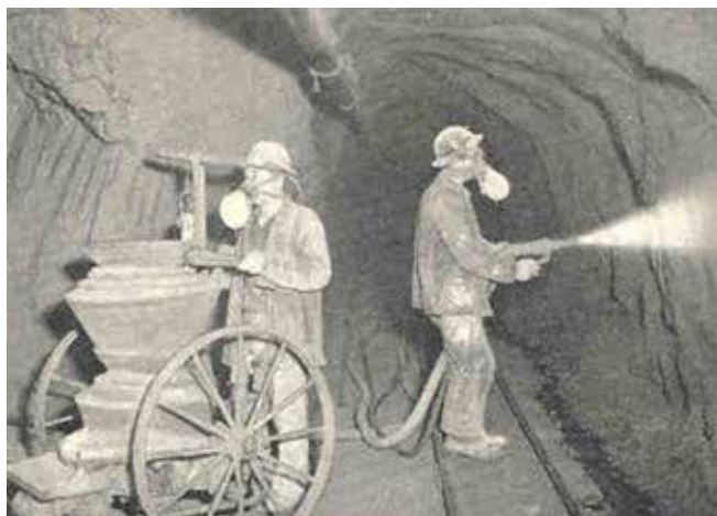
Fig. 2: Lining a tunnel with gunite using a double-chamber gun in the 1920s
