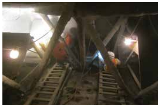
Fig. 2 and 3: Shotcrete placement inside the arches
