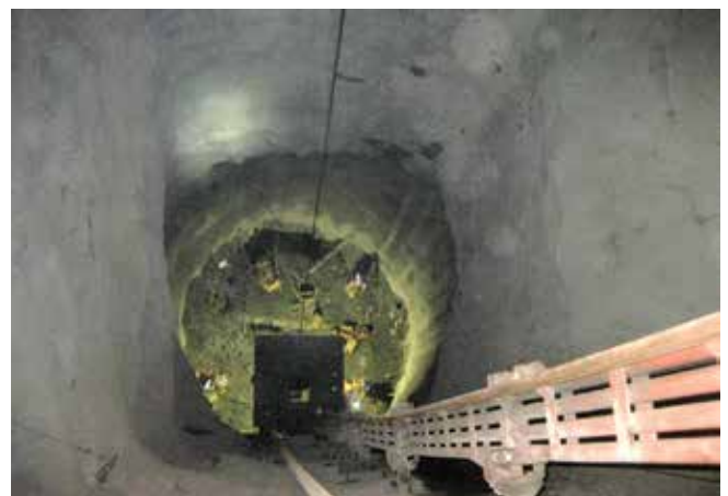
Fig. 3: Construction and installation of protective shotcrete lining for critical ore pass in a Northern Quebec gold mine
