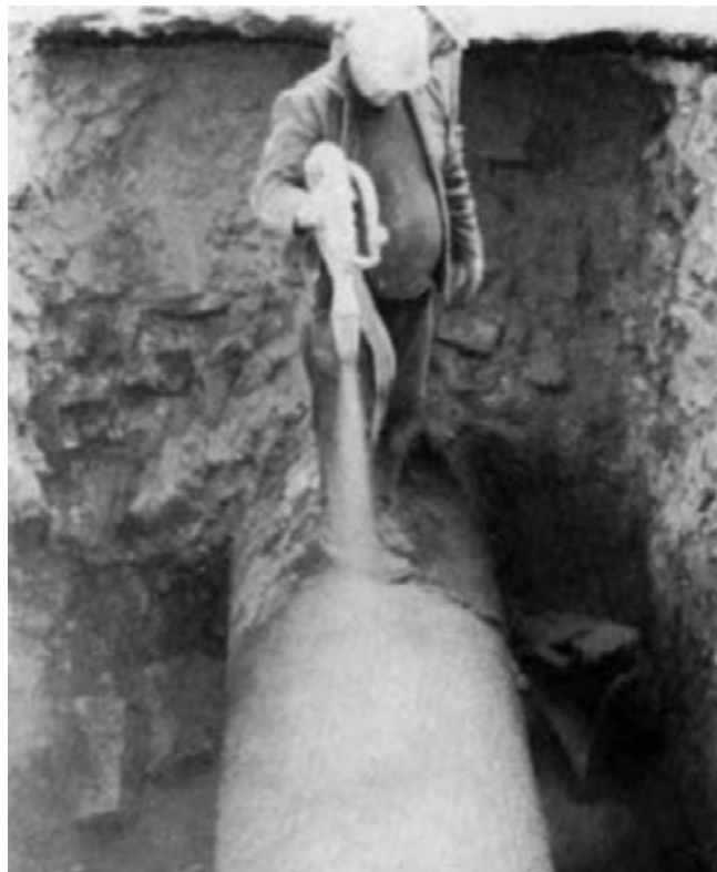
Another wide-spread use of shotcrete is for the protection of pipe from corrosion. It is also often used to coat the interior joints of mortar-lined pipe
