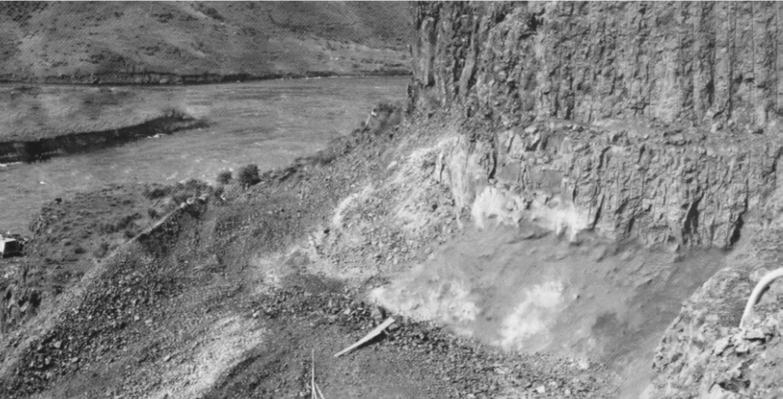
Figure 1. Rock slope stabilization with SFRS, Snake River, Idaho, 1972
