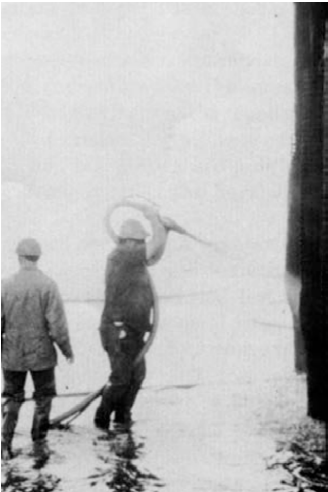
Shotcrete being applied over existing wood piling that had considerable erosion damage. By use of mesh-reinforced shotcrete, the pier was salvaged and is back in use
