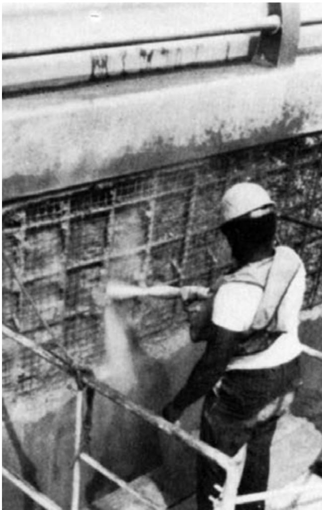
Wetting down an area prior to shotcreting
