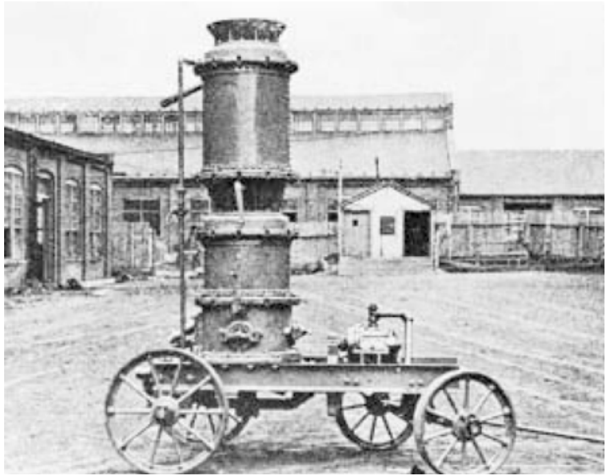
The original machine used in 1907 to recoat the facade of the Field Museum of Chicago. (Photo courtesy of J.J. Shideler, Portland Cement Association, Skokie, IL)
