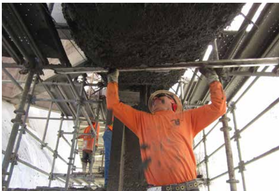
Fig. 8: Overhead finishing
