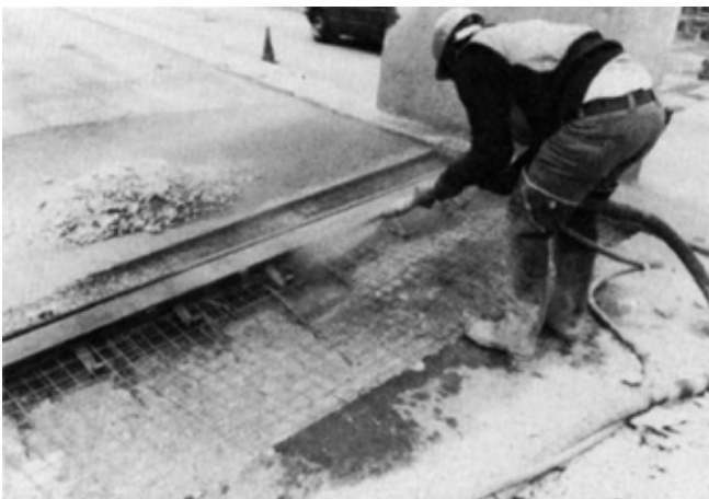
Shotcrete expansion dam became loose, had to be rewelded
