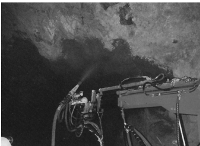
Figure 6: Manipulator arm application of SFRS in Deep Copper Shaft at Mt. Isa Mines, Queensland, Australia
