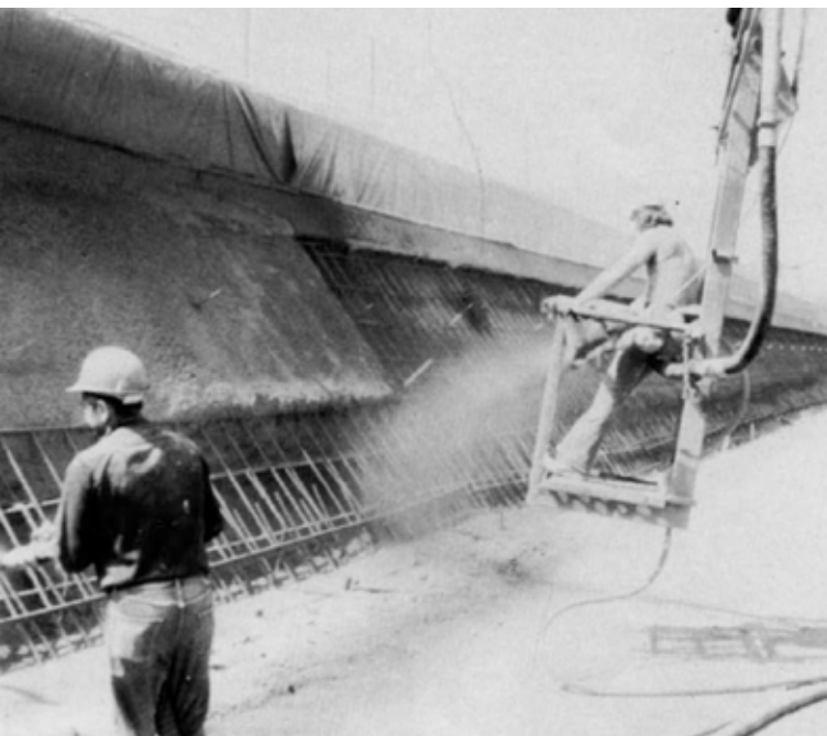
Shotcrete is often placed from a boom bucket as well as from grade level
