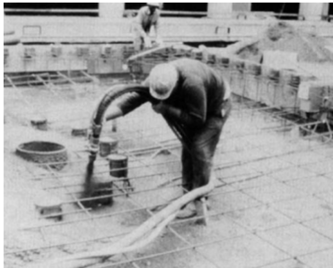
Water-jetting equipment from a fountain is being encased in air-placed concrete. The nozzleman is directing the stream around this equipment to ensure proper imbedment
