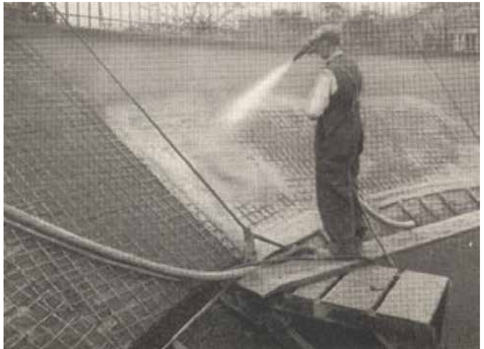
Figure 2. Nozzleman applying "Guniting" for a water storage facility in Pittsburgh, 1919
