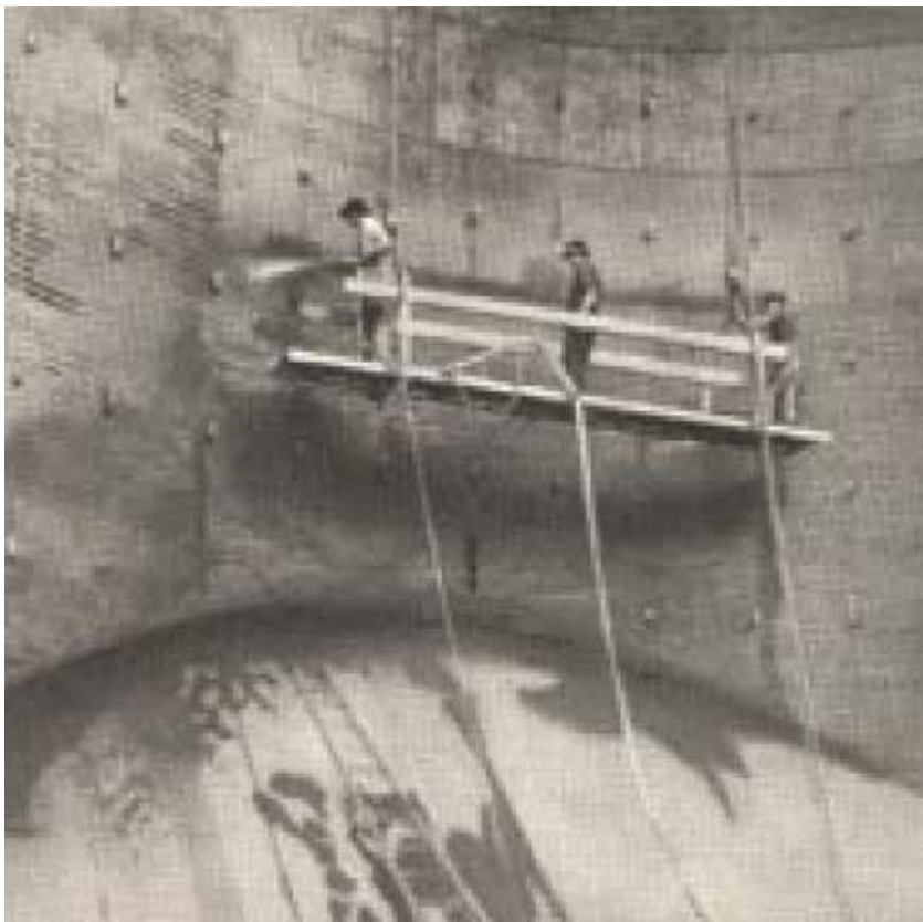
Figure 3. Restored, reinforced "Gunitite" flue at American Smelting and Refining Co., Helena, Montana, 1924
