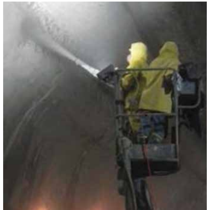
Fig. 2: Application of macro-synthetic fiber shotcrete in the Billy Bishop Pedestrian Tunnel 5
