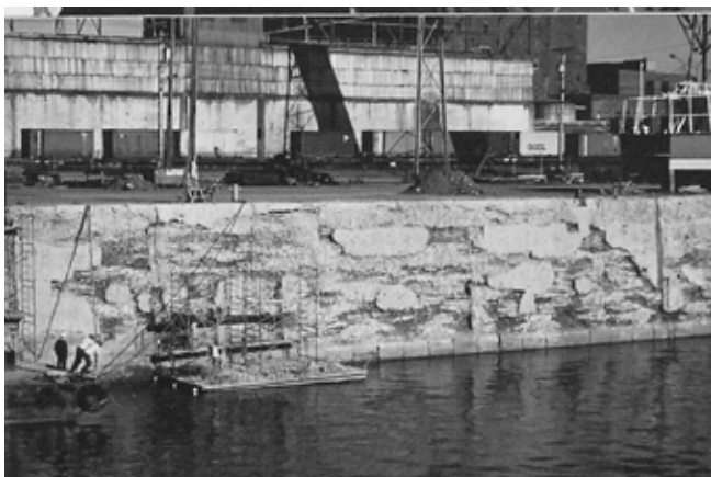
Figure 5: Preparation of shipping berth faces at Port of Montreal, Quebec, Canada
