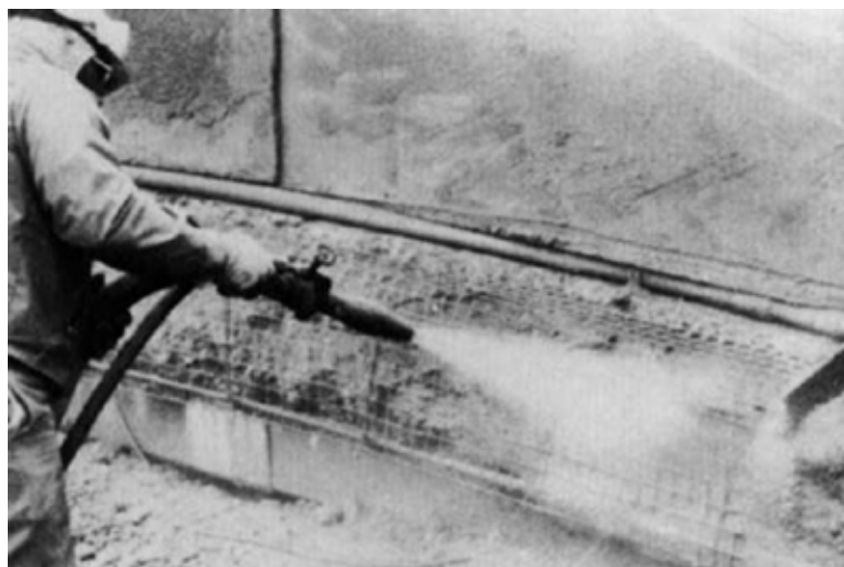
Shotcreting fascia beam; area to right is overshot
