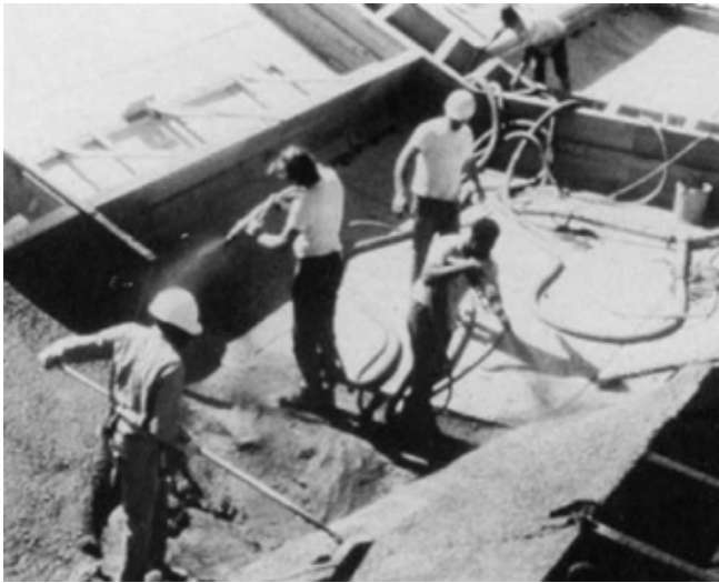
Because of the high compaction density achieved by air placement, finishing operations can start immediately
