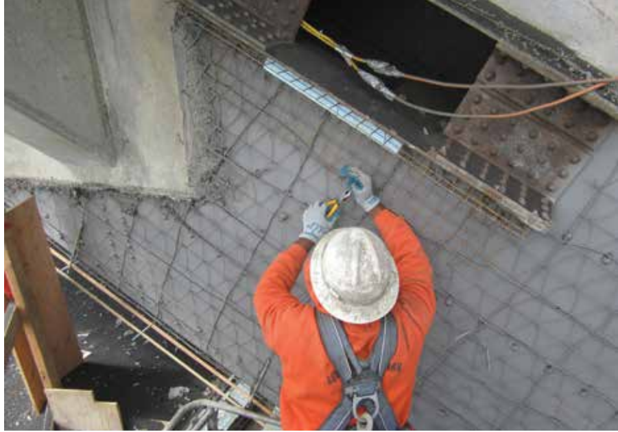
Fig. 4: Repairing mesh prior to shoot
