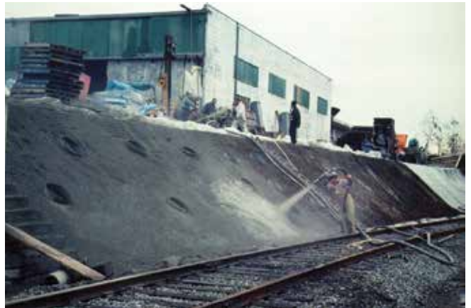
Fig. 4: Dry-mix steel FRS lining of a railway embankment in Burnaby, BC, Canada, in 1978
