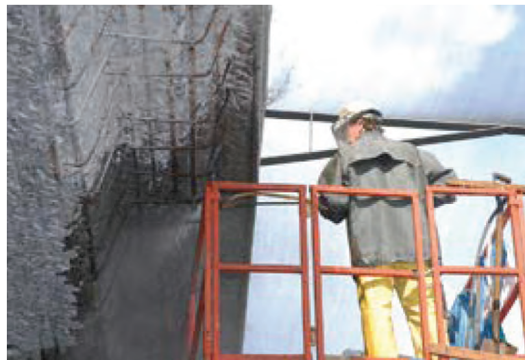
Fig. 3: High-pressure cleaning of the prepared concrete substrate prior to shotcrete application
