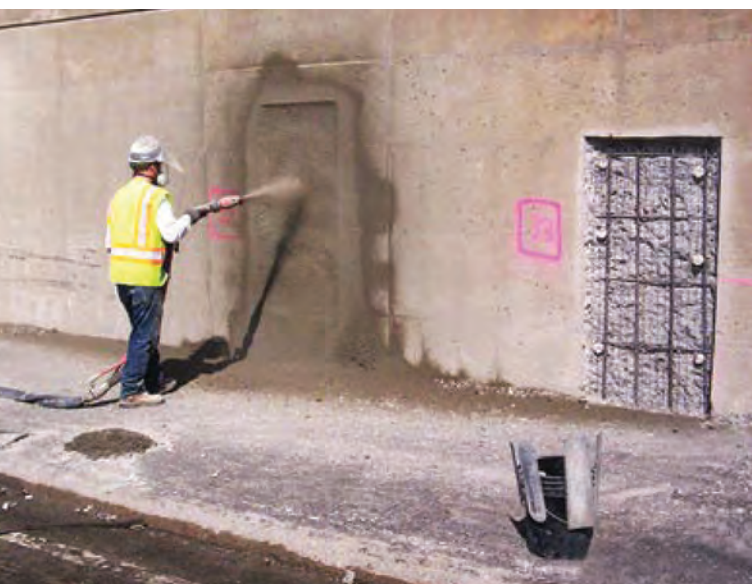
Fig. 1: Concrete (shotcrete) pneumatically projected at high velocity to repair area
