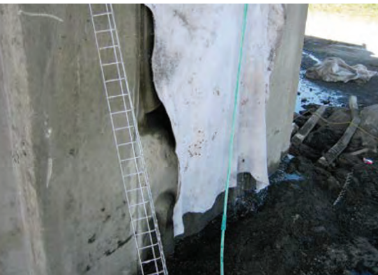
Fig. 5: Wet curing must be continuous for a minimum period of 7 days.
