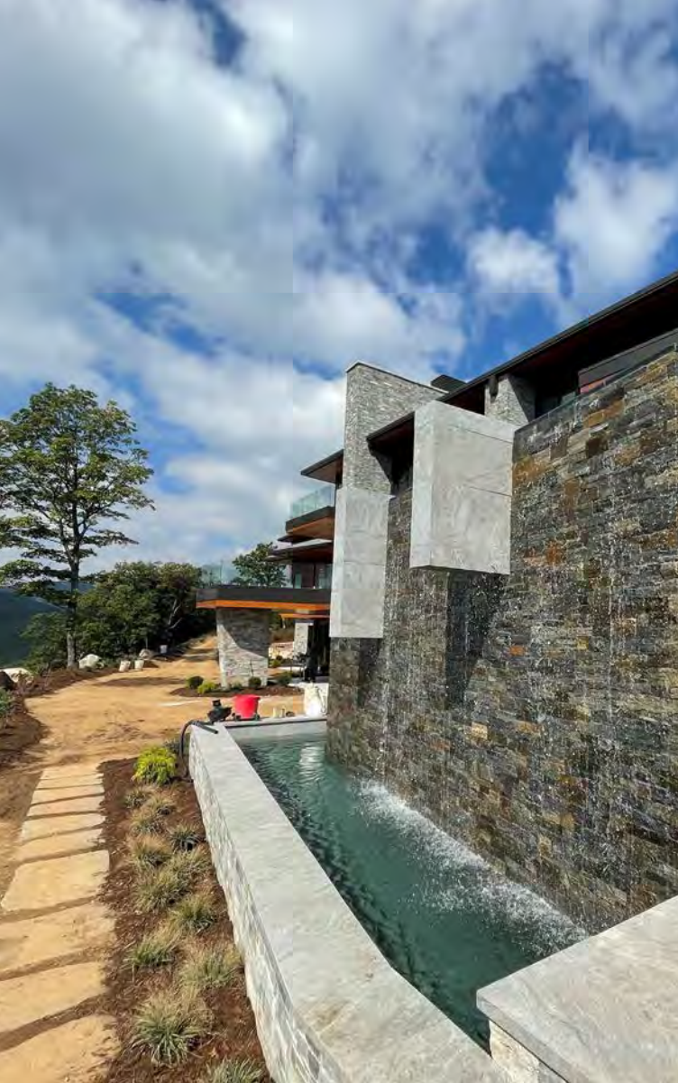
Fig. 11: Intersecting planes shot in place with pool shell
