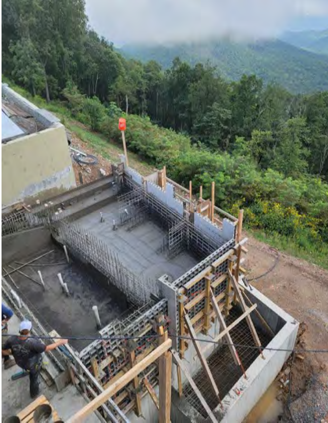
Fig. 2: First the pool floor was shot along with a gutter wall, which allowed the forming of the shelf and additional bar
