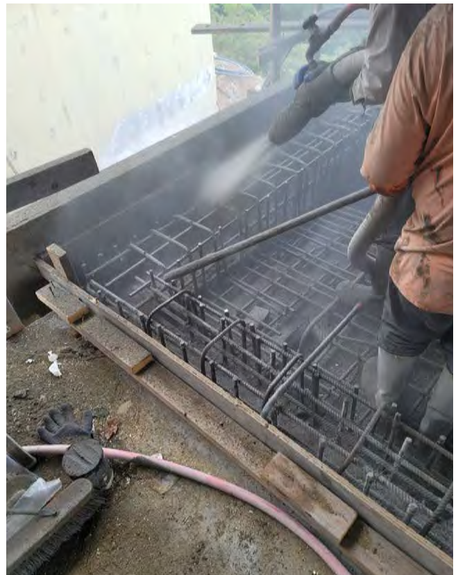
Fig. 4: Air lance operator keeping the corner free from rebound until the nozzleman places material in the corner. High quality diaphragm water valve ensures a sensitive control of mix water
