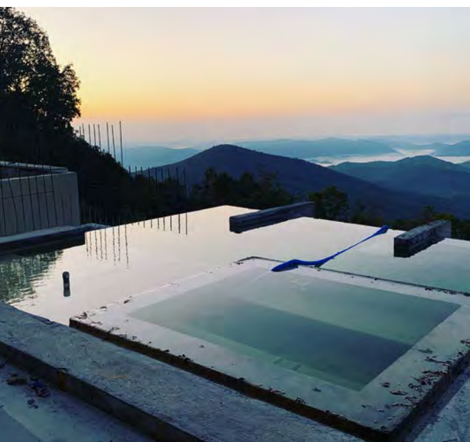
Fig. 12: Water Curing shell by flooding the project
