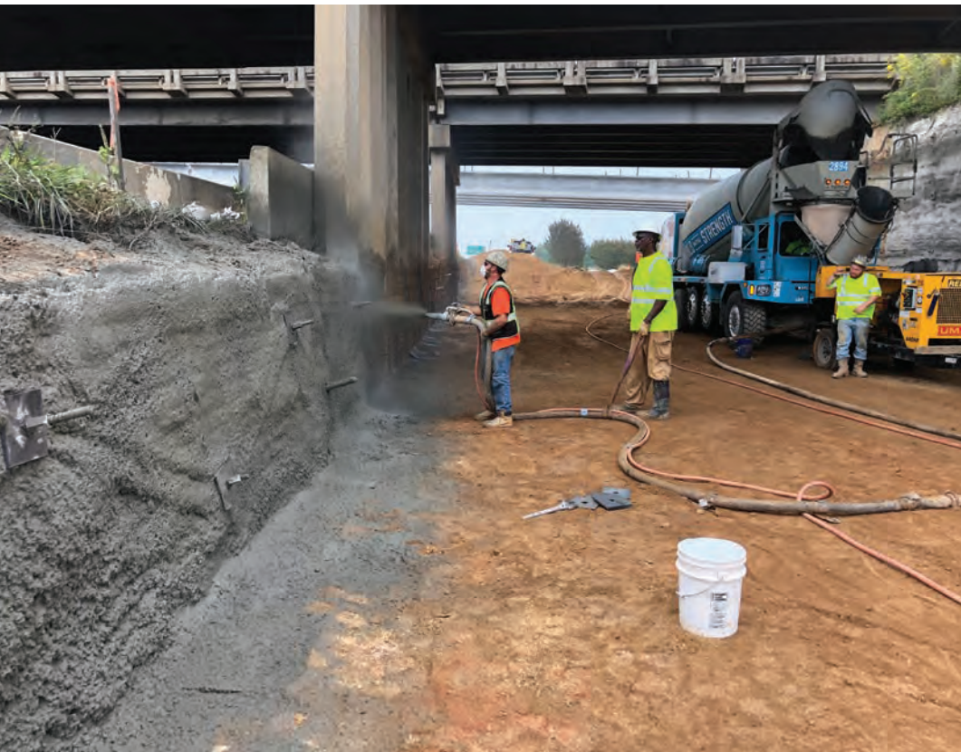
UMA's earth retention and sculpted shotcrete work on NCDOT's I-40/I-77 interchange improvements project held up cuts for widened roadway sections and facilitated new bridge construction.
