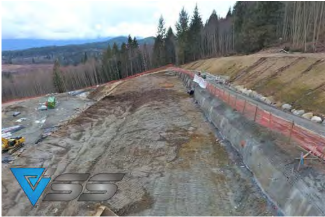
Fig. 2: Beginning of project
