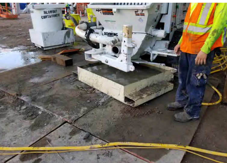
Fig. 7: Off-site project mock-up with final eggshell coating system
