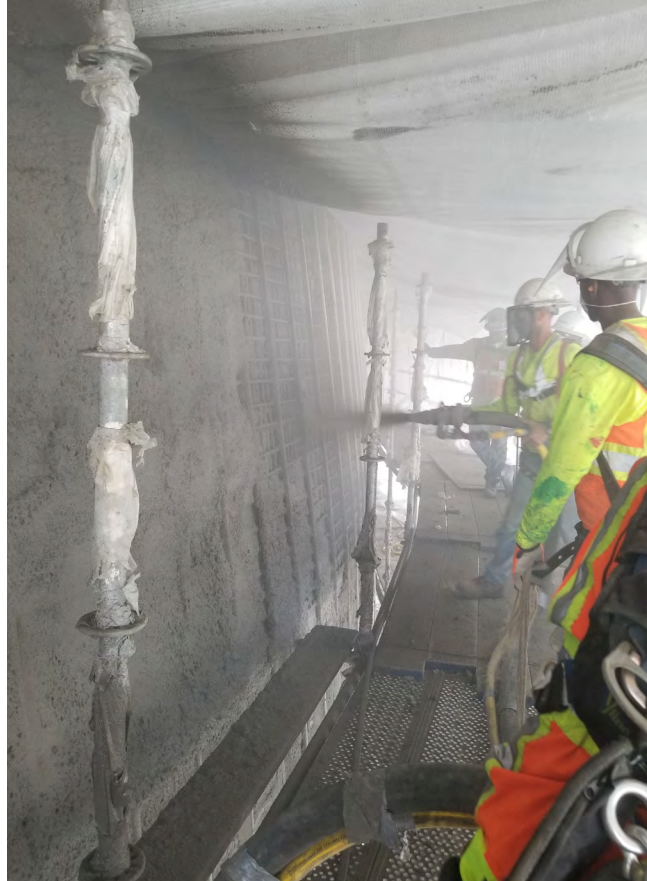
Fig. 9: Shotcrete application, note extensive containment to control overspray and protect surrounding structures
