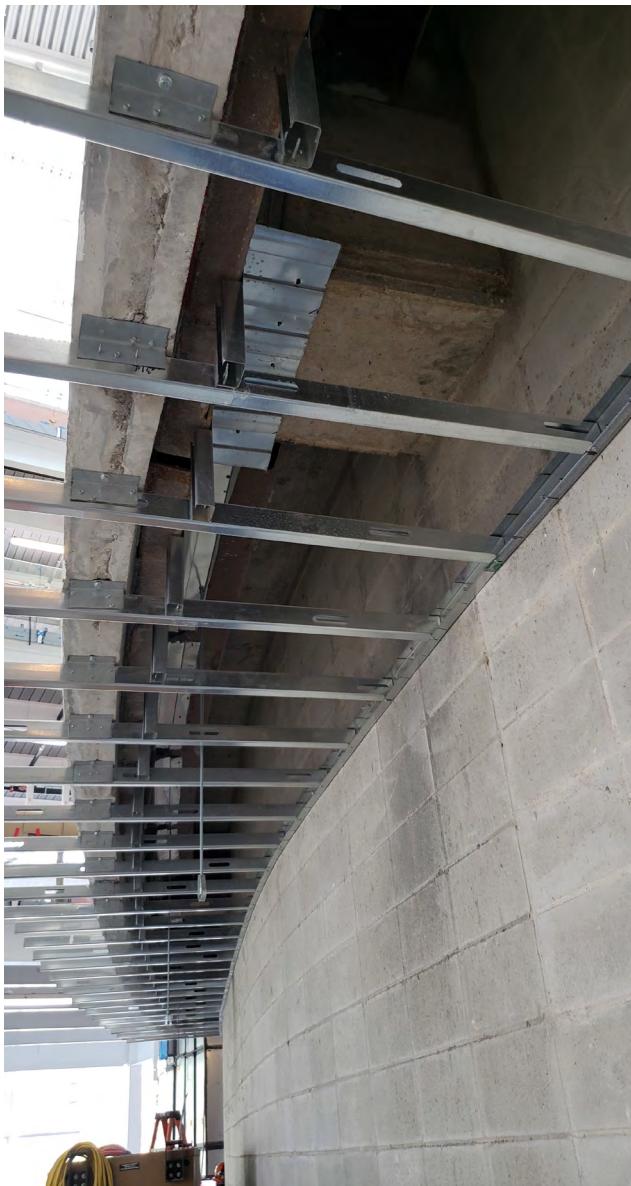
Fig. 4: Tubular structural steel framework and reinforced cast-in-place concrete columns and beams
