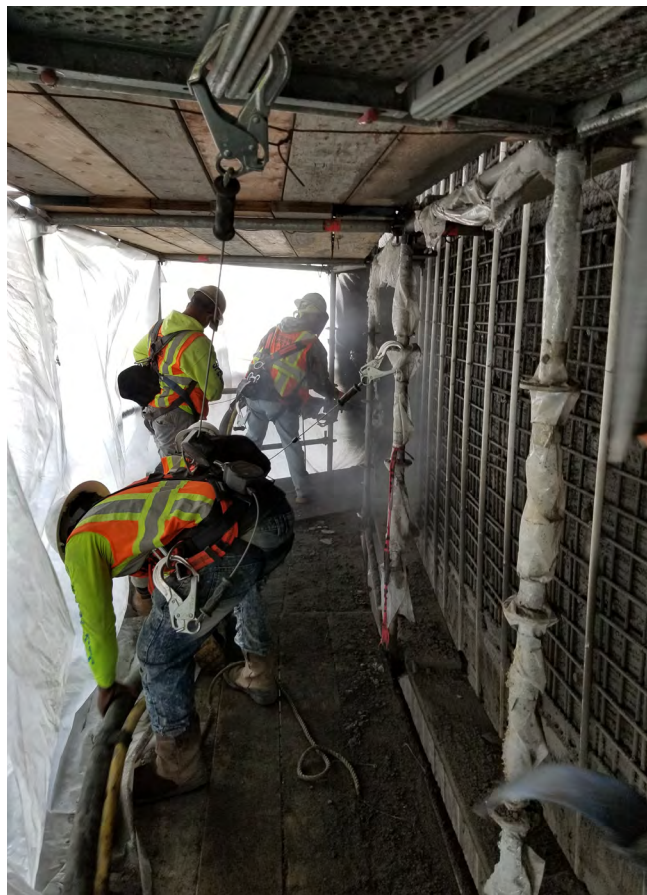
Fig. 10: Extensive containment measures taken to control overspray and protect surrounding structures during shotcrete application
