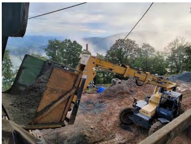
Fig. 7: Rebound removal
