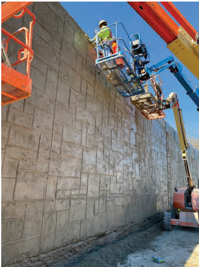
Craftspeople in man baskets performed all sculpted shotcrete work by hand, from spraying material to carving the artistic patterns.
