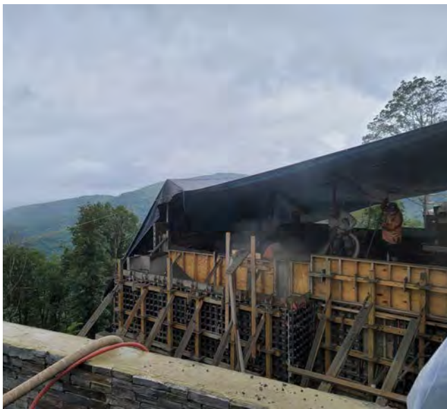
Fig. 3: Rain protection with a tarp. Nozzlemaster with an air lance operator at his side, keeping the adjacent material clean. Complex forming
