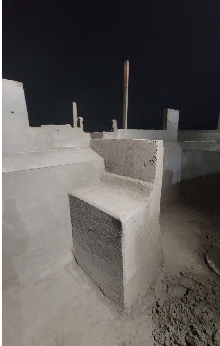
Fig. 9: Intricate shapes can be placed and finished in one shoot
