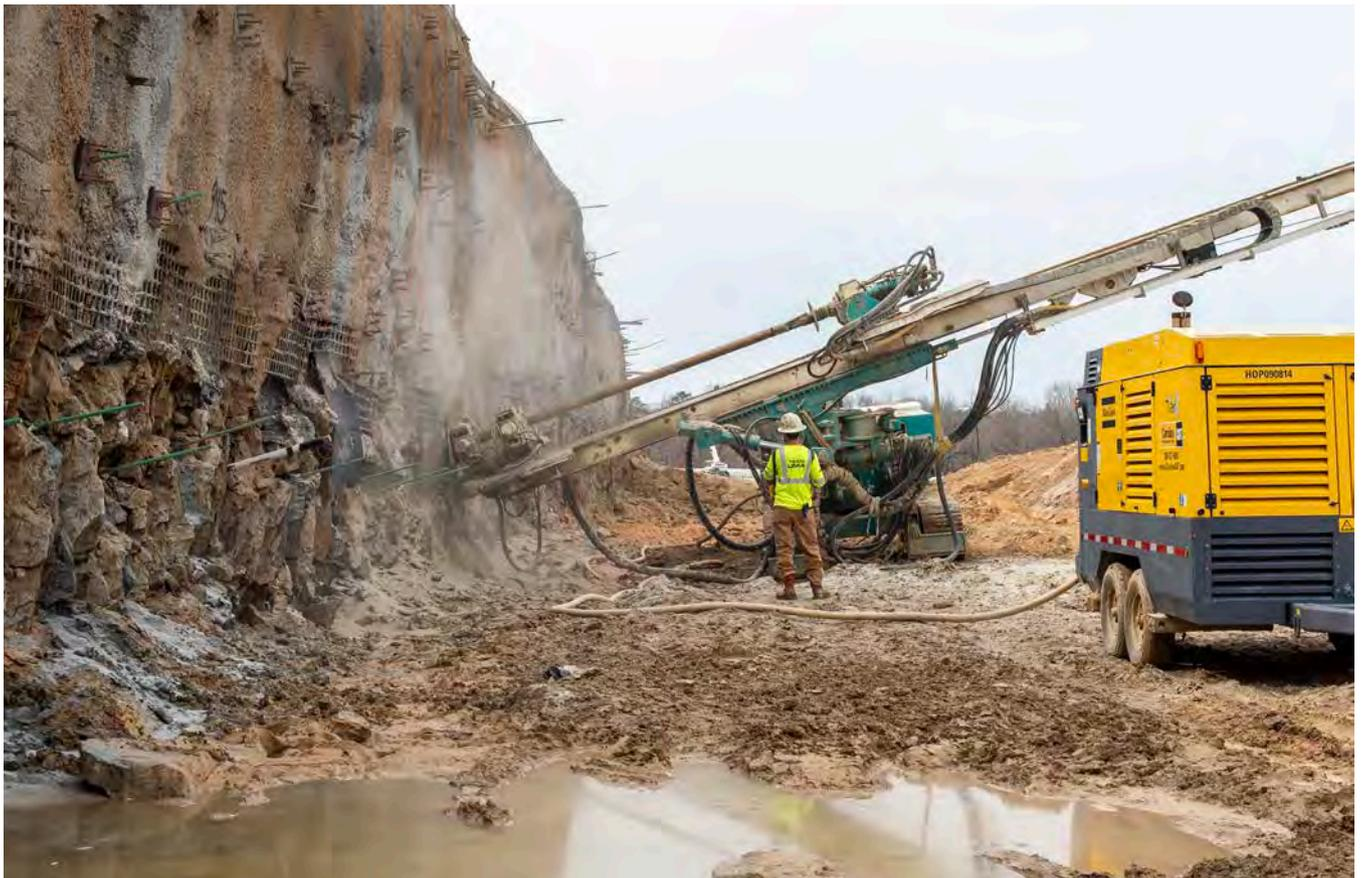
UMA Geotechnical Construction's work on the NCDOT I-26 Exit 40 to I-40 Interstate Expansion Project is on track to become the largest square footage of soil nail walls done under a single contract in NCDOT history.
