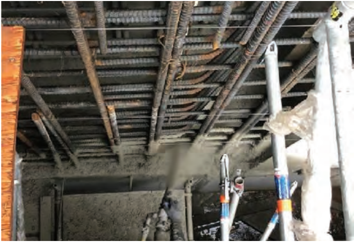
Fig. 12: Guide wires installed to control wall thickness and finishing. View from top deck. Shooting started at corner of wall.
