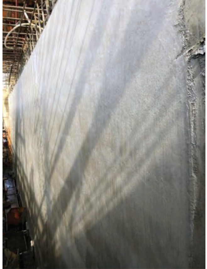
Fig. 23: View of shotcrete wall surface from second deck; no thermal cracking was observed.
