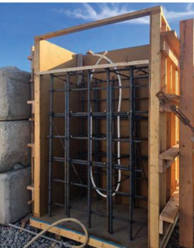
Fig. 2: Mockup for mass concrete wall with two layers of 25M reinforcing bar and cooling pipes.
