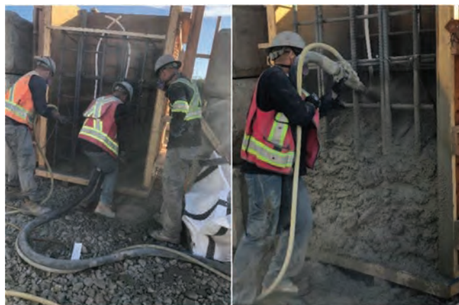
Fig. 4: Shotcrete construction of mockup wall.
