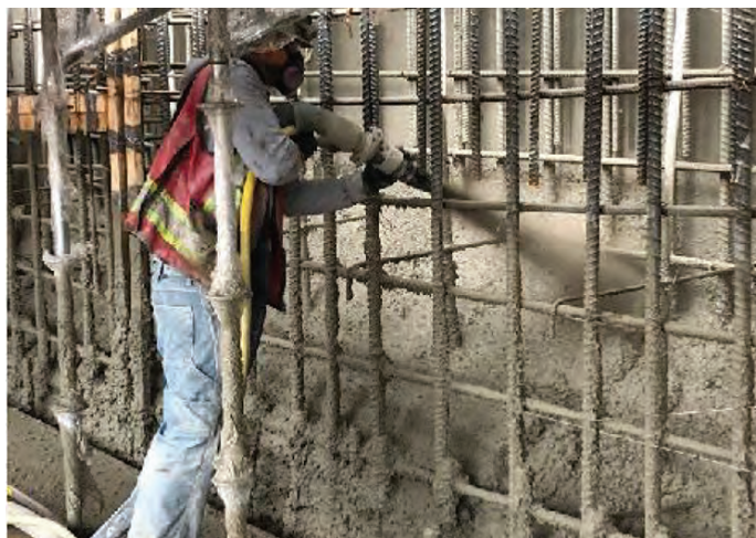
Fig. 15-Nozzleman moved nozzle into 300 x 300 mm reinforcing bar grid to fill up back layer of reinforcement. Note that nozzle angle was kept at approximately 90 deg. to receiving surface. Note that guide wires were used to control thickness of wall, and were cut and removed after finishing.
