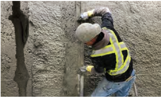
Fig. 19: Screeding finish coat to guide wires.
