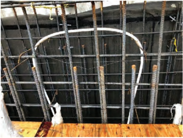
Fig. 13: Cooling pipe installed at 1.0 m spacing with four inlets.
