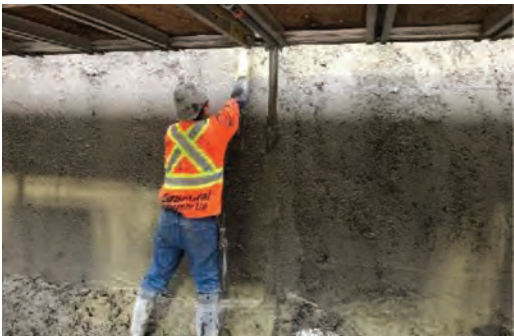
Fig. 20: Float finishing with darby.
