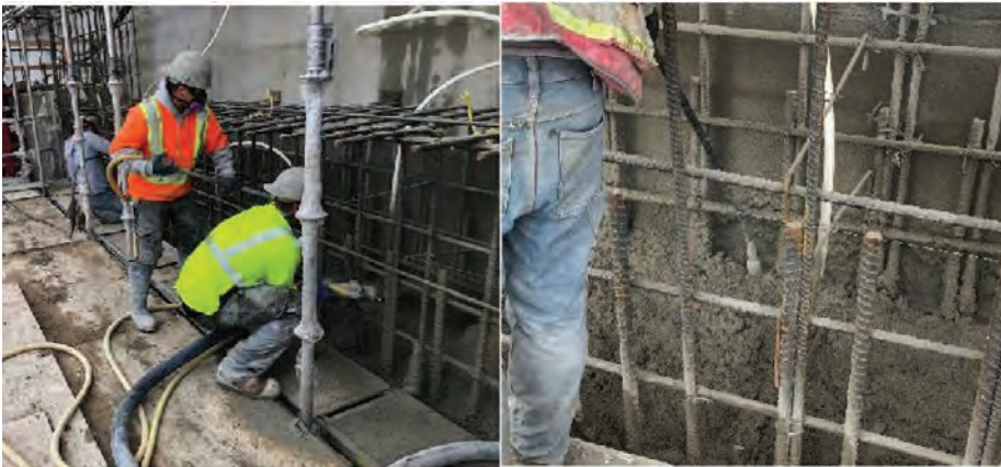
Fig. 17: Shooting, blow pipe operation, and light touch with pencil vibrator to enhance final consolidation.
