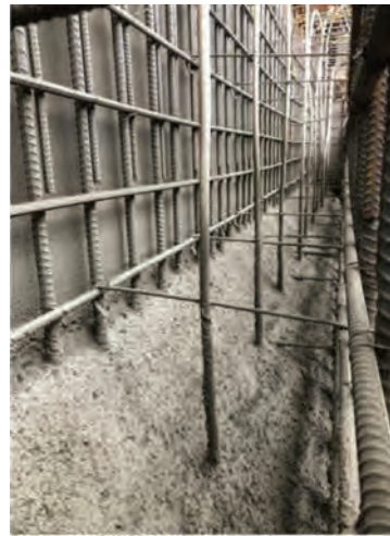
Fig. 16: For each lift, shotcrete was applied to approximately 45-deg. slope. Prior to application of next lift, rebound and overspray were removed by blow pipe.
