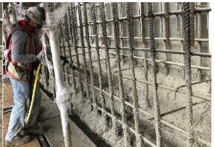
Fig. 15-Nozzleman moved nozzle into 300 x 300 mm reinforcing bar grid to fill up back layer of reinforcement. Note that nozzle angle was kept at approximately 90 deg. to receiving surface. Note that guide wires were used to control thickness of wall, and were cut and removed after finishing.
