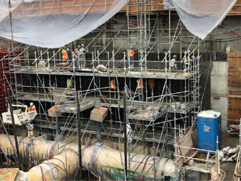
Fig. 10: View of scaffold (three-deck platform), shotcrete crew, and finishing crew with tarp on top to protect wall from rain.
