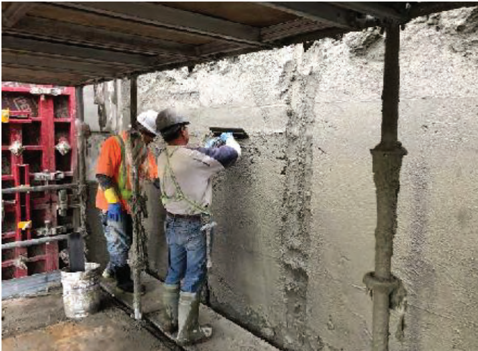
Fig. 21: Final steel-trowel finishing.
