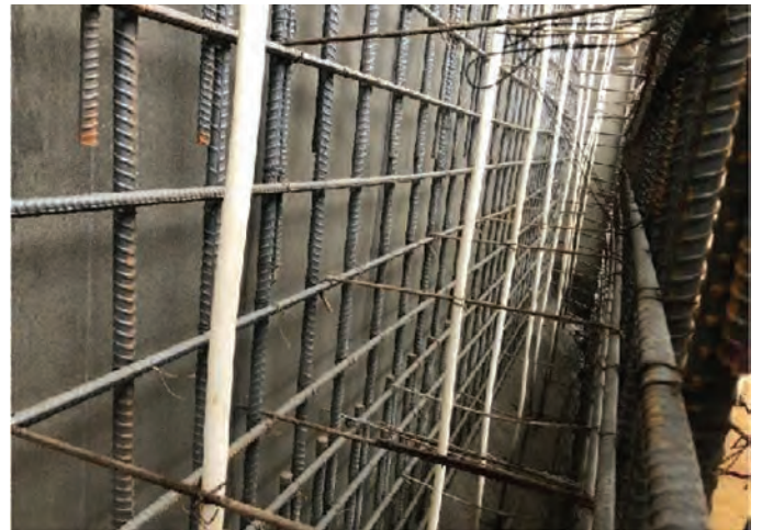
Fig. 11: Two layers of 25M reinforcement with cooling pipes (fixed using tire wire with auxiliary 10 m stirrups) erected in middle thickness of wall.
