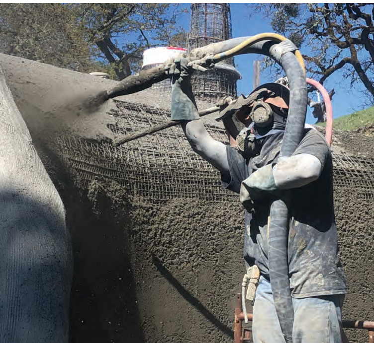
Fig. 2b Note clamping of the tip hose with arm.
