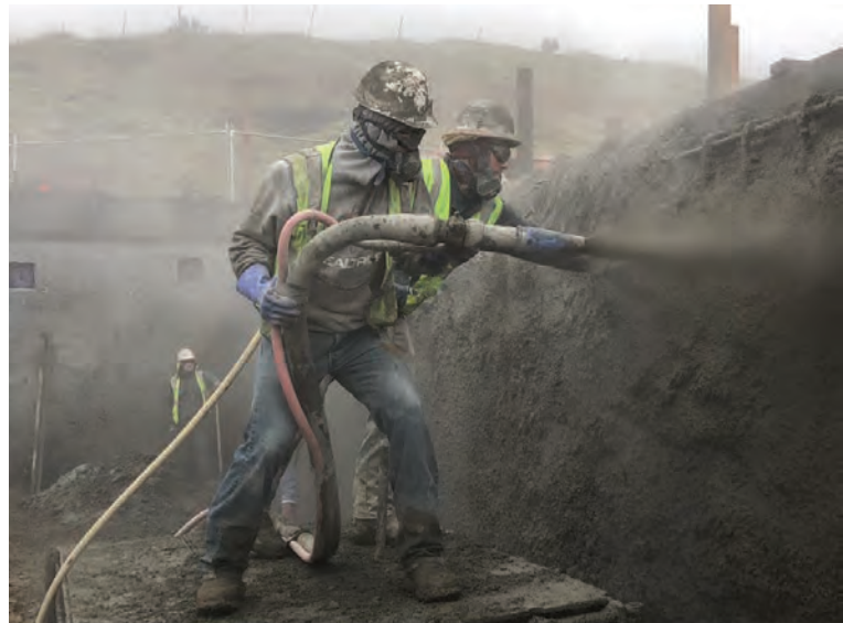
Fig. 2a The hose is placed on the ground and arced upward by the nozzleman's legs. The tip hose must be sufficiently rigid to continue its upward arc
