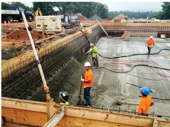
Fig. 1: Floor cast with installed keyway
