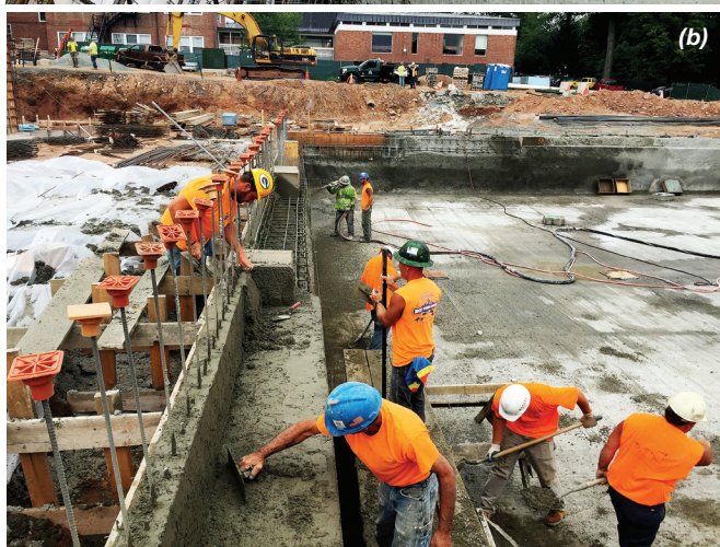
Fig. 2(a) and (b): Shotcrete on top of cast floor
