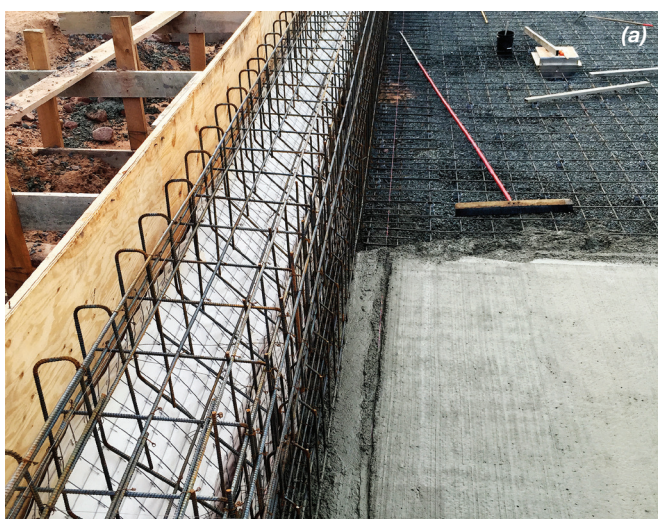
Fig. 1: Floor cast with installed keyway
