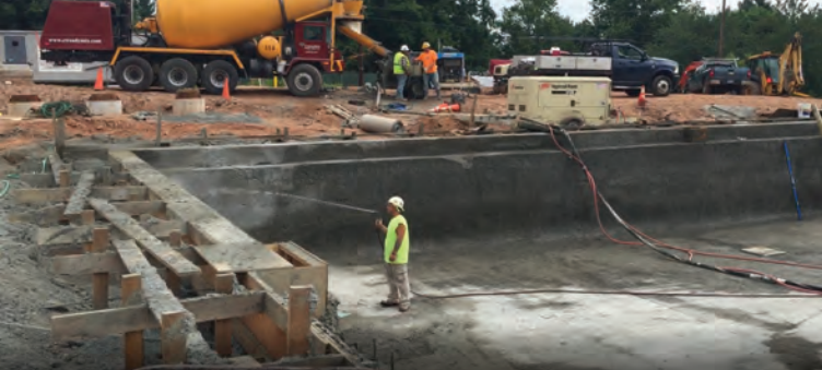
Wetting down freshly shot walls after finishing
