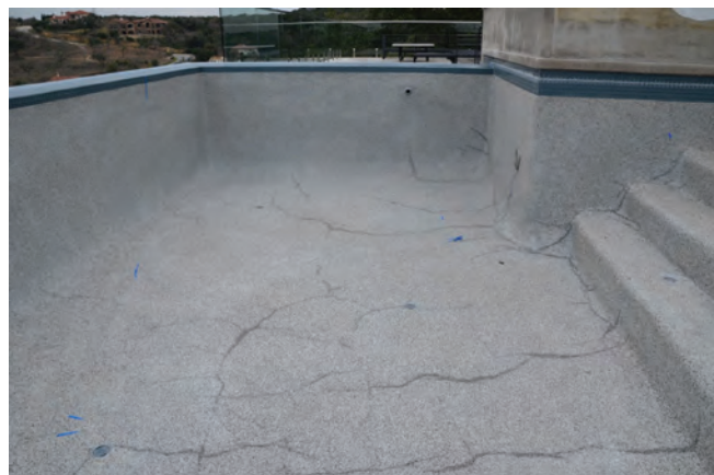
Cracking in the concrete pool shell from inadequate curing will mirror through the plaster coating.
