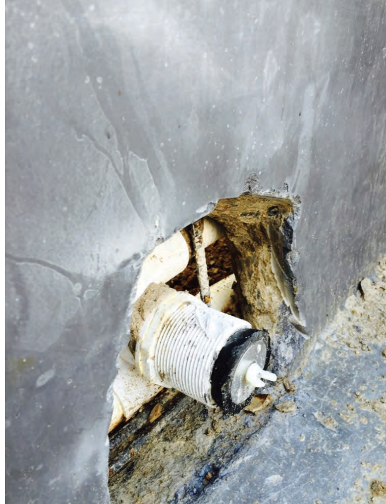
Fig. 2: Thin wall shotcrete, insufficient concrete placement and no encapsulation of surrounding penetrations or steel reinforcement
