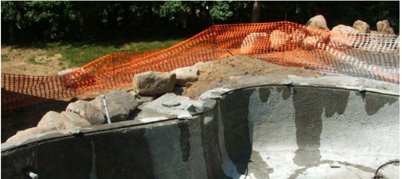
Partial wetting is not acceptable. All exposed concrete must be kept continuously wet for 7 days.
