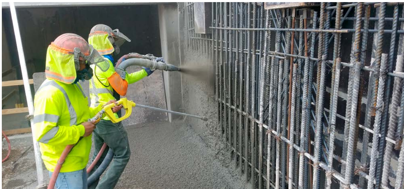
Shotcrete operations with compliant air gun.
