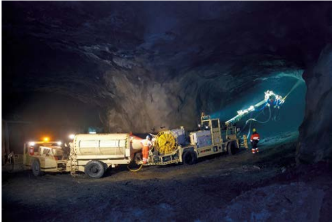
Fig. 6: Typical setup showing concrete hauler (left) feeding concrete pump of mechanized sprayer (right).
