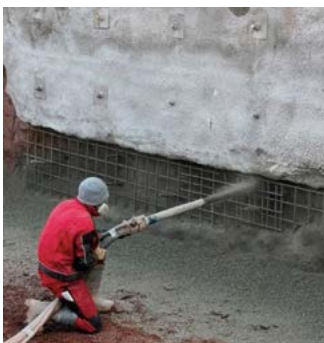
Fig. 1: Shotcrete application by hand.
