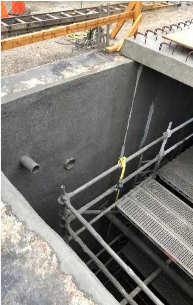
(#19M) bars at 6 in. (150 mm), an application of shotcrete (KPM Industries MS-D1) to restore the wall profile to original thickness, and lastly the application of the protective polyurea coating system.
