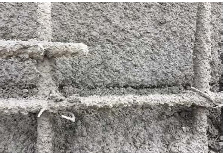
Fig. 6a. Tracking occurring within the shadow area is easy to see. Tracking behind reinforcements is visual evidence that the mixture is far too stiff.
