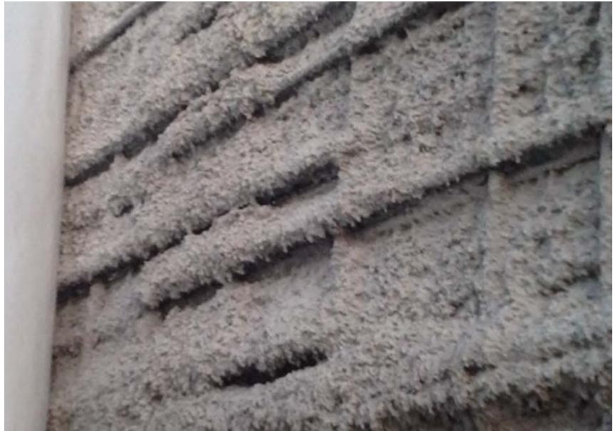
Fig. 5. Visual evidence of buildup on the reinforcement was ignored by the nozzleman. Note the massive voids that have formed behind the bars.
