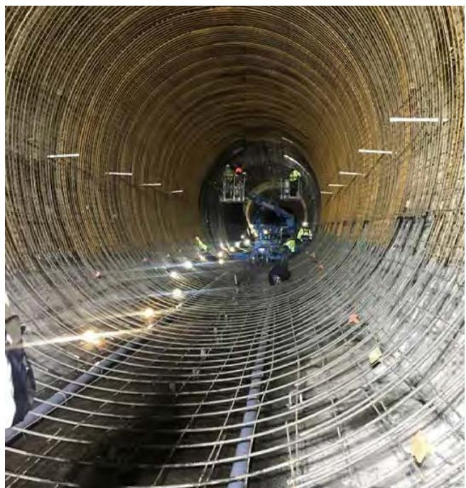
scheduled to begin. The tunnel design thickness was 10 in. (250 mm) thick, not including overbreak and other repair work. The final shotcrete volume installed was over 500 yd<sup>3</sup> (380 m<sup>3</sup>).
