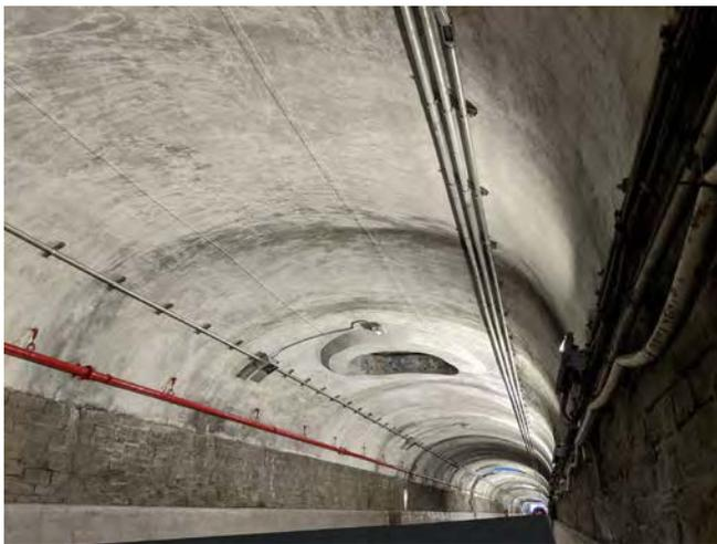
been. Since shotcrete placement eliminated the need for erection and removal of complicated formwork, the owner enjoyed significant cost savings due to reduction of both labor and materials. Additionally, the elimination of formwork reduced the overall embodied carbons consumed throughout the project's lifespan.
