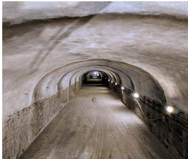
applied to the previous day's work. This served as the finishing lift, allowing for the use of less set-accelerating admixture, meaning the crew had more time to perfect the sponge float finish. Cruz mixed, applied, and finished approximately 25 to 30 yd<sup>3</sup> (19 to 23 m<sup>3</sup>) of 3 in. (75 mm) slump concrete material per day.
