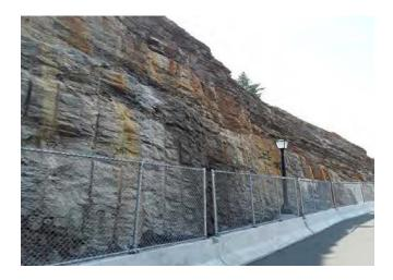
The wall behind the barracks, which was exposed to a combination of exposure to the sun, as well as freezing and thawing, caused the rock to become weathered and brittle. This created the need for our work, because without an engineered solution the exposure would continue to erode the mountain side. The US Army Corps of Engineers (USACE) were tasked to provide a solution for this extensive exposed rock wall face. An elaborate sculpted shotcrete system was the answer.
