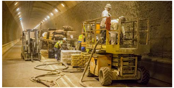
PennDOT Liberty Tunnel wall rehabilitation, Pittsburgh, PA
