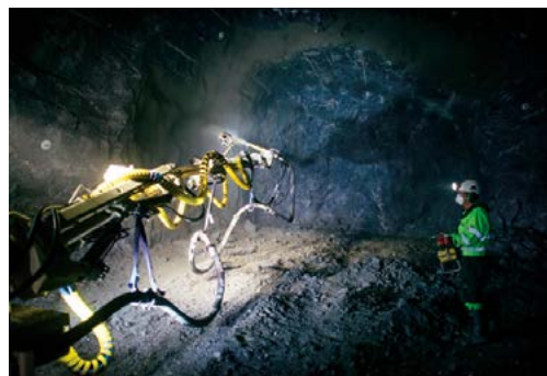
Fig. 2: Shotcrete application by mechanized equipment via radio remote.
