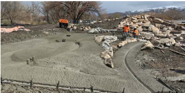
Fig. 2: Ground support shotcrete placement benefited from the two nozzles
