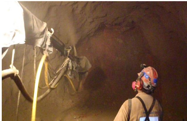
Fig. 2. Shotcrete placement with a remotely operated nozzle
