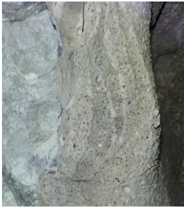
Fig. 4. Good bonding between shotcrete layers
