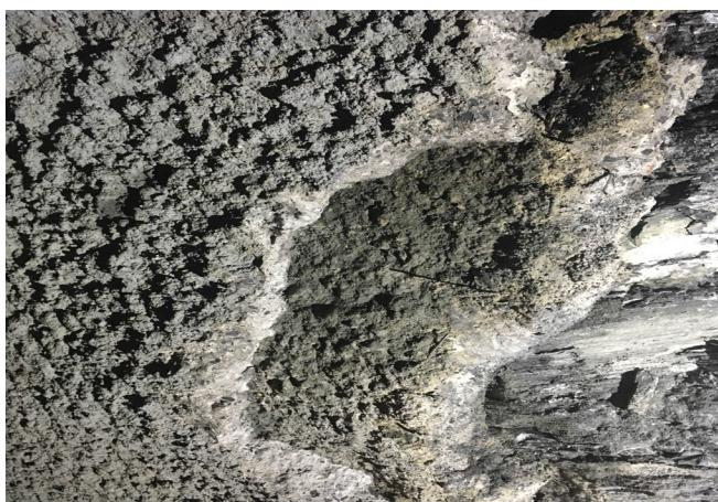
Fig. 3. Lack of surface preparation prevented adhesion between concrete layers and concrete and rock.
