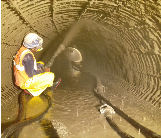
Fig. 9: Placing wet-mix shotcrete
