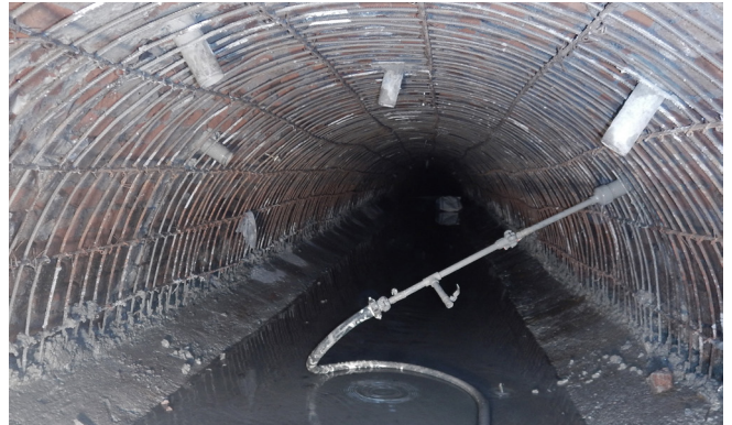
Fig. 11: Fixing injection packers and grouting using a non-shrink cementitious, anti-washout grout
