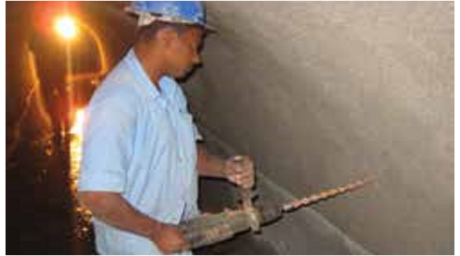
Fig. 10: Drilling holes into the brick masonry
