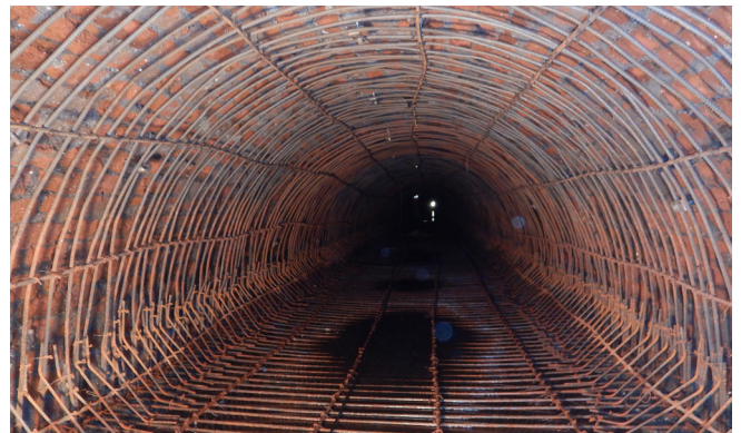
Fig. 8: Fixing steel reinforcement
