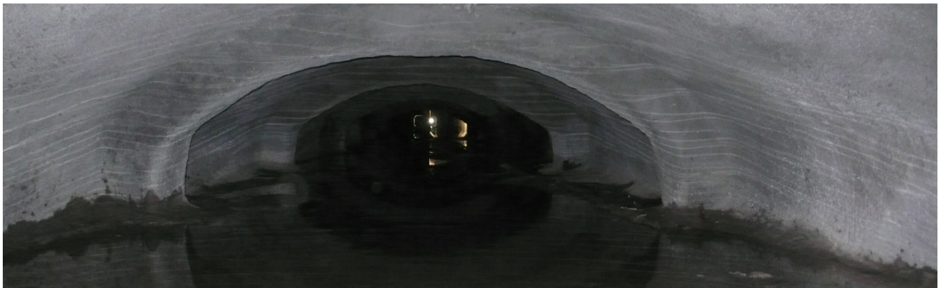
Fig. 1: Completed repair of the storm water drains in the City of Mumbai, India, that are over a century old and were constructed of brick arch masonry during the British Era
