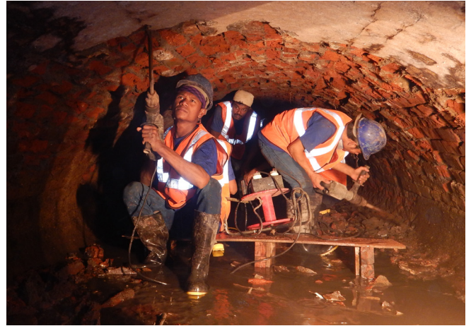
Fig. 5: Demolition of deteriorated brick lining with lightweight breaker
